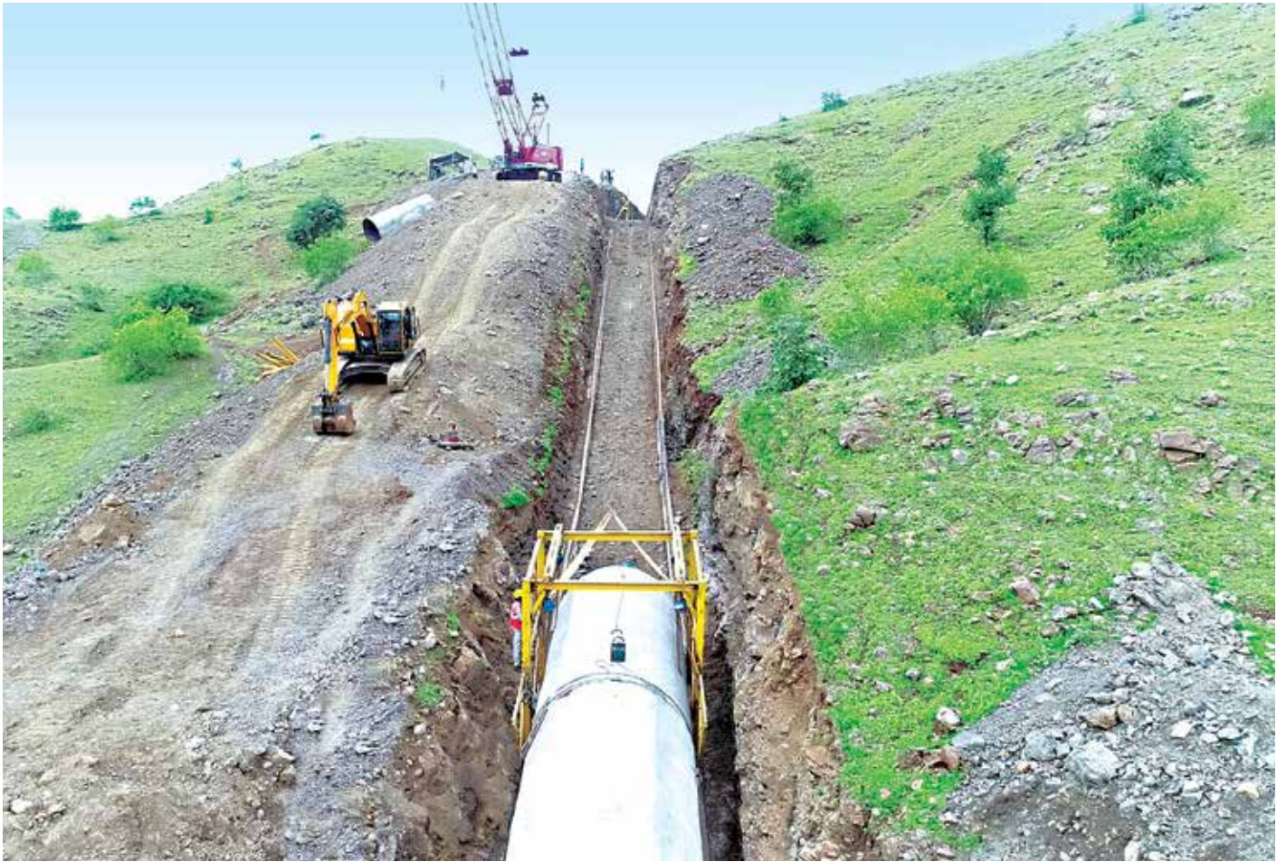
Winch and trolley system for shifting and laying MS pipes at Alirajpur MLIS Project
