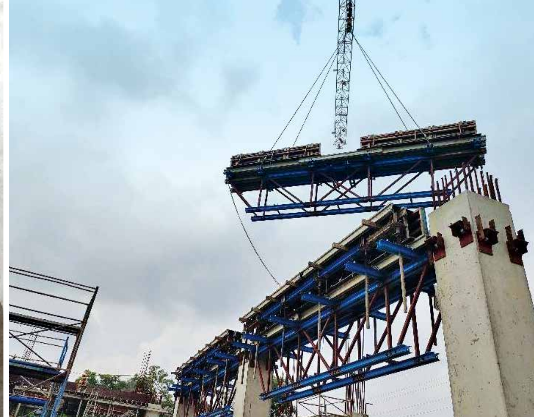
Fly table erection
