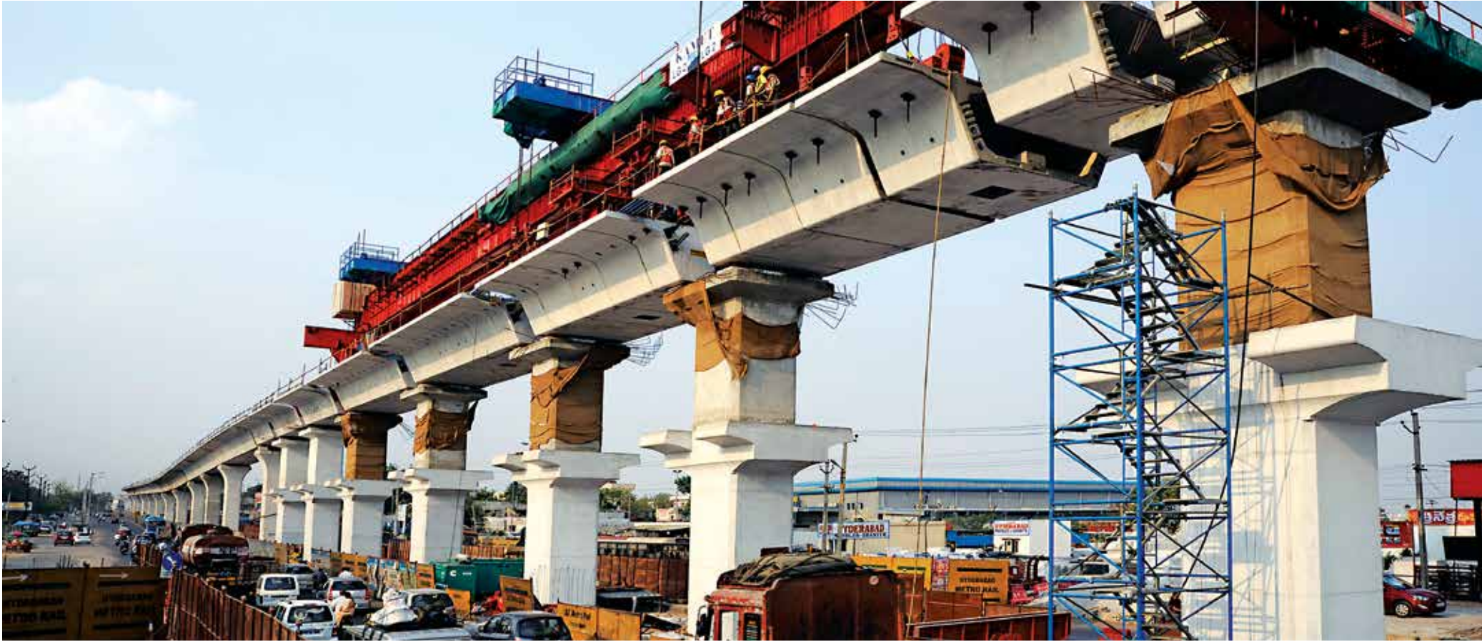
Girder erection at Hyderabad Metro Rail Project
