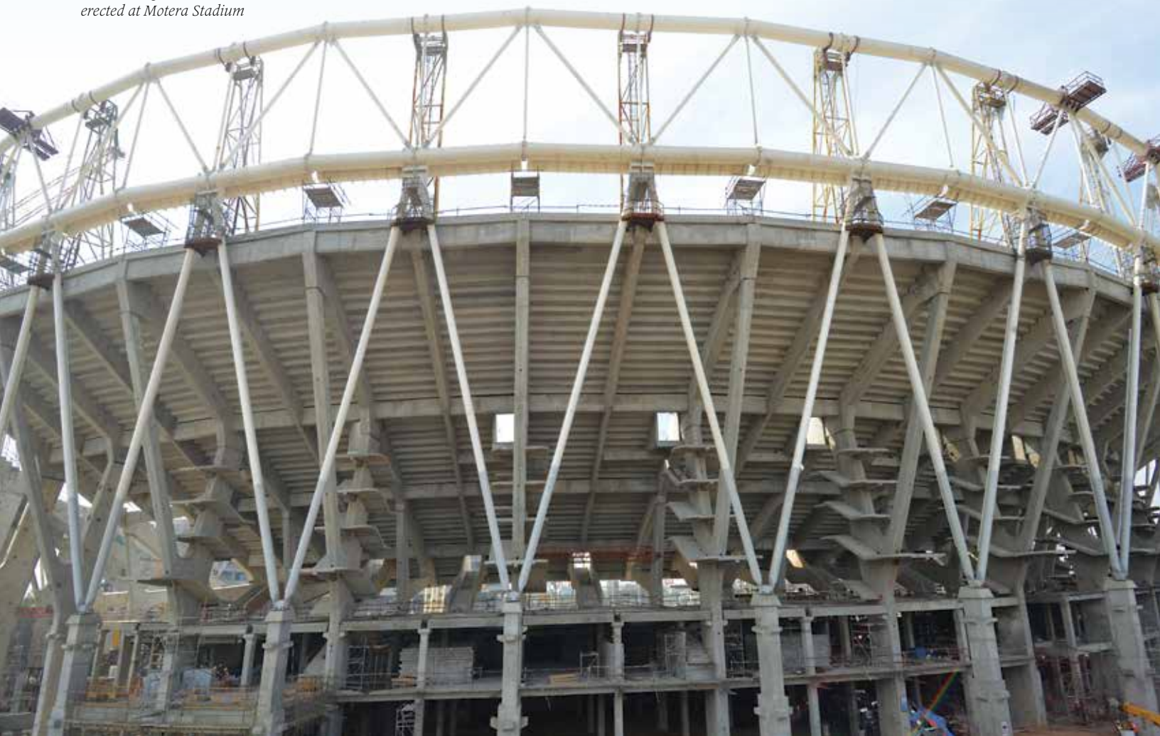
GY and HY precast columns erected at Motera Stadium
