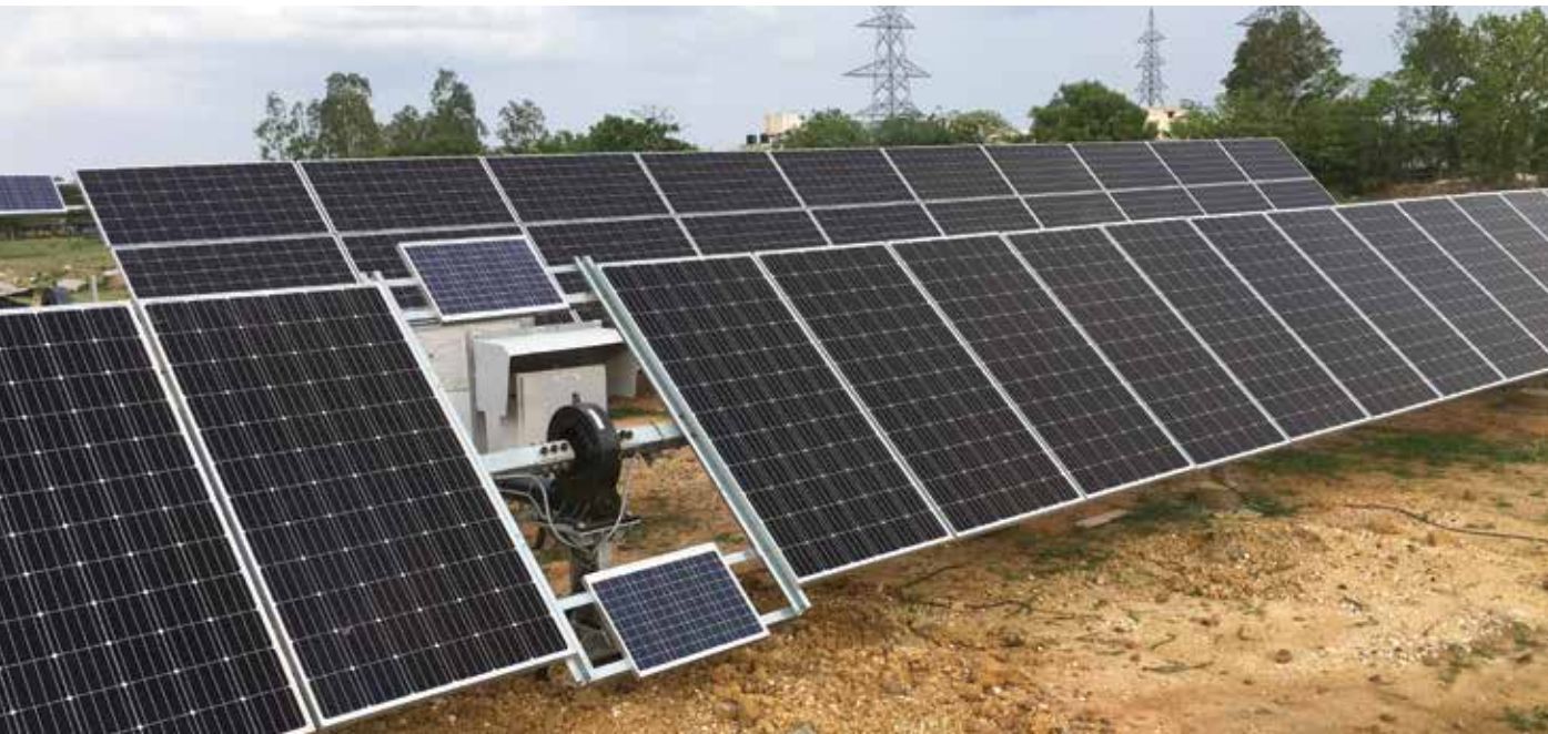
Single axis tracker block and single row tracker variants
