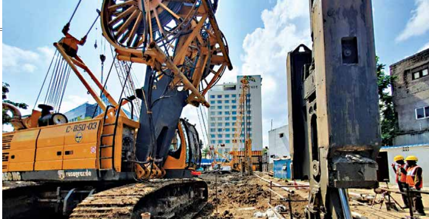
Diaphragm wall works for a project in Chennai
