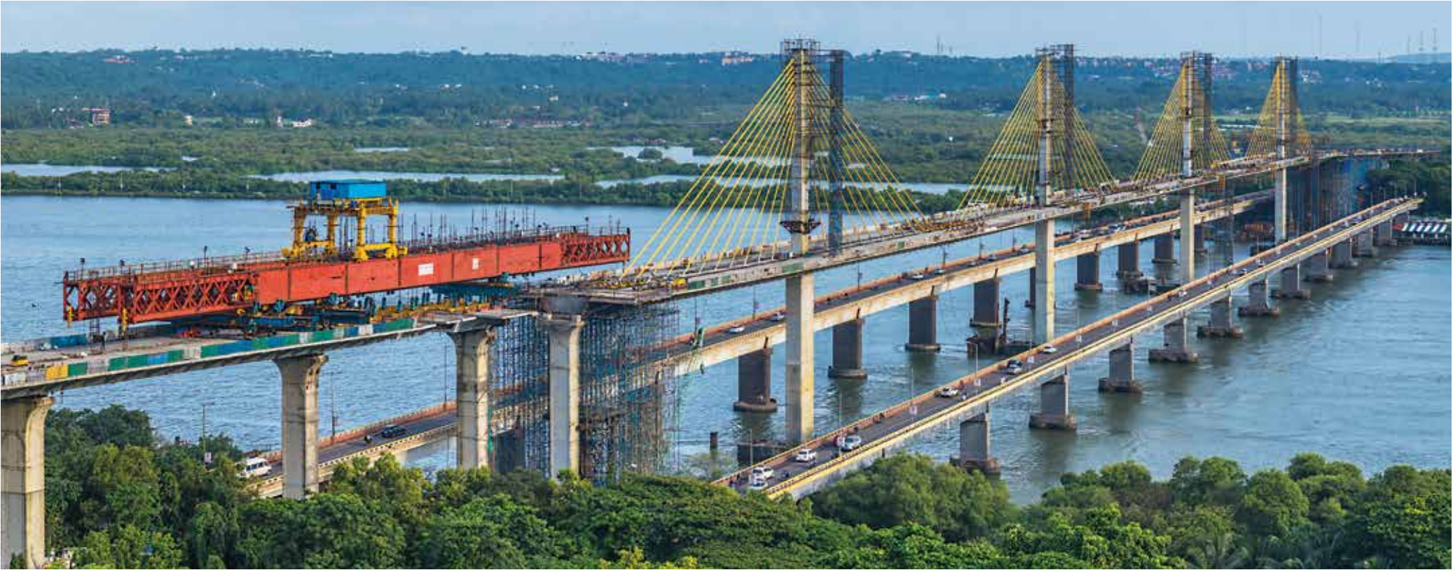
Launching girders at Mandovi Bridge Project
