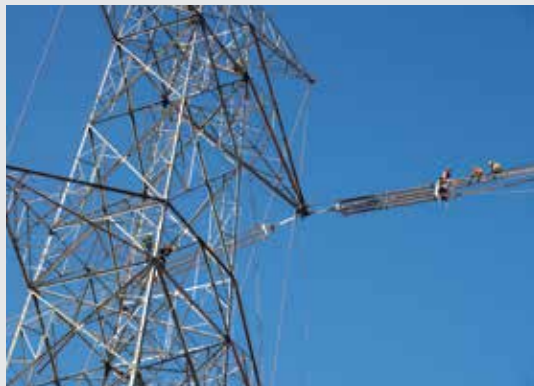
Workmen on lifelines to raise the steely tower members
