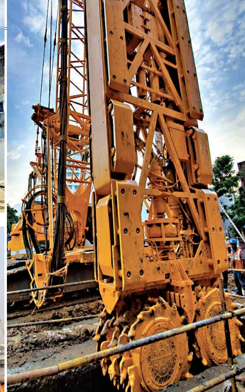
Trench cutter in action
