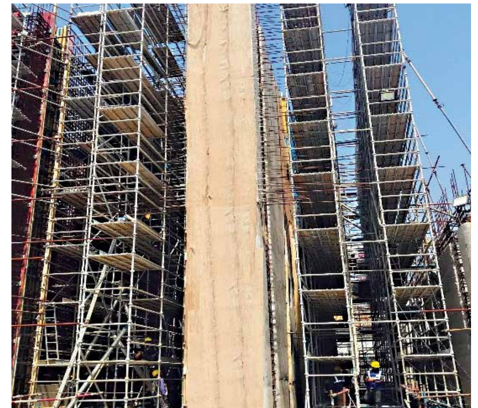
16-meter tall formwork system for Kudankulam Nuclear Power Plant
