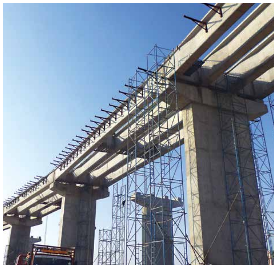
Precast girders installed for fast tracking the construction of an elevated corridor
