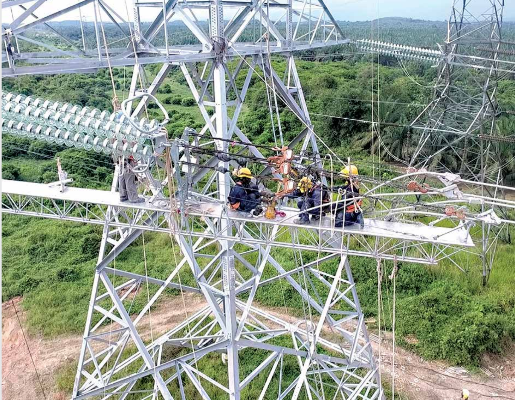
A safe platform on sag bridges for transmission tower erections
