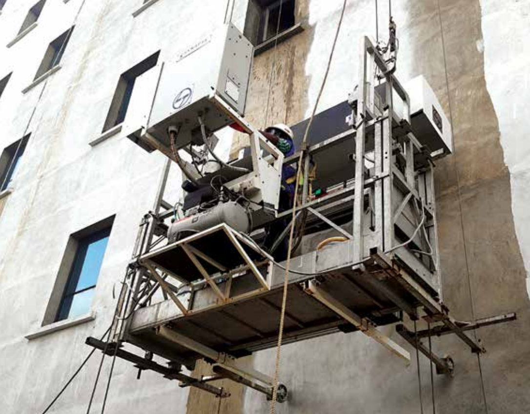
External wall robotic painting
