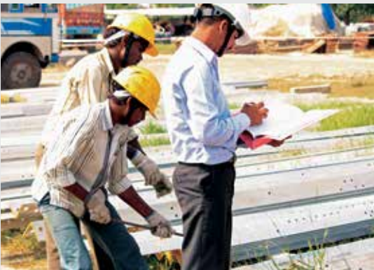
Tagging of transmission tower members
