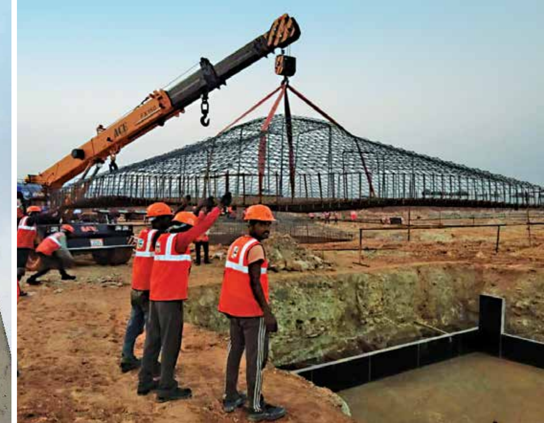
Rebar Reinforcement Cage
