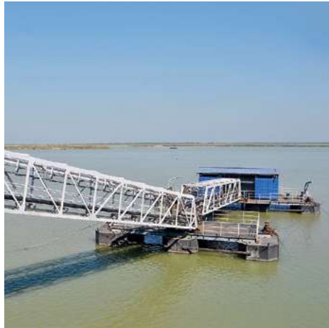
Floating barge intake, Sahibganj, Jharkhand
