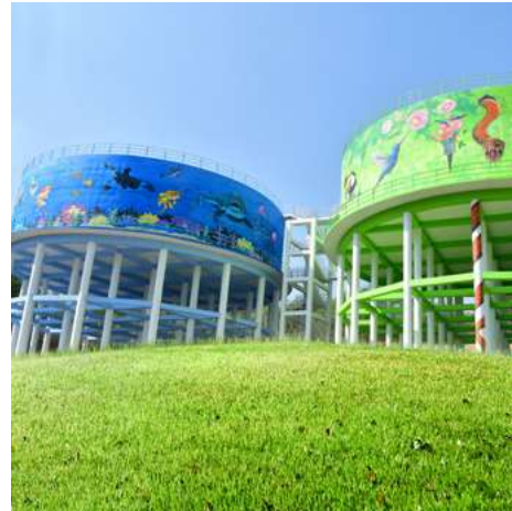
Elevated Storage Reservoir, Pune, Maharashtra
