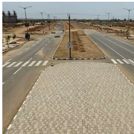
Green-field development at Dholera, Gujarat
