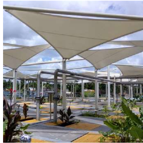
31 MLD Wastewater Treatment Plant, Bhatpara, West Bengal
