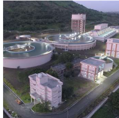
137 MLD Water Treatment Plant at Nashik, Maharashtra
