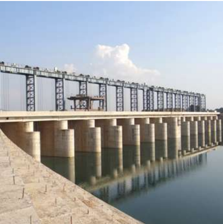
Kharkai Barrage, Jharkhand
