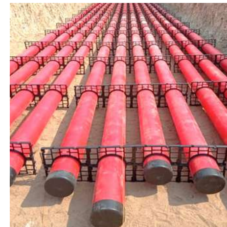
PLB Duct at Amaravati, Andhra Pradesh
