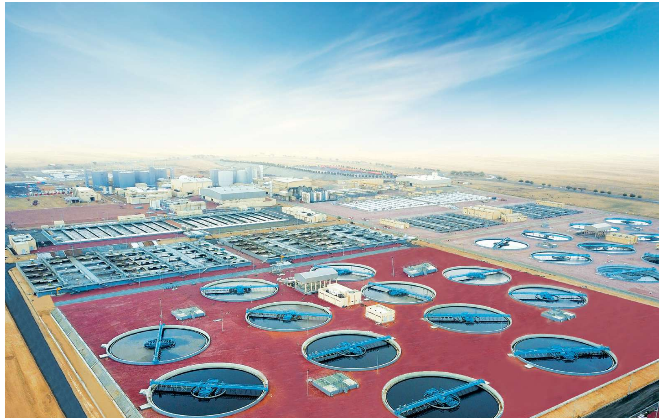
375 MLD Wastewater Treatment Plant, Jebel Ali, UAE
