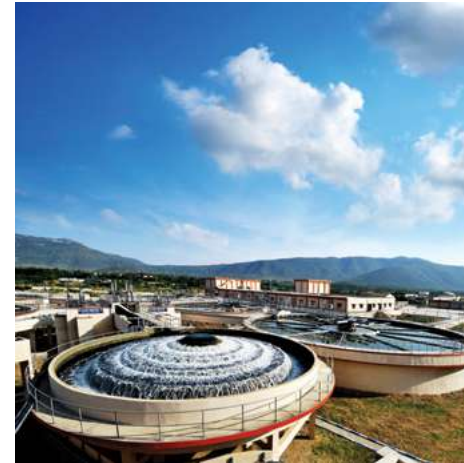
181 MLD Water Treatment Plant, Vellore, Tamil Nadu
