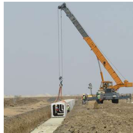
Precast duct laying at Amaravati, Andhra Pradesh
