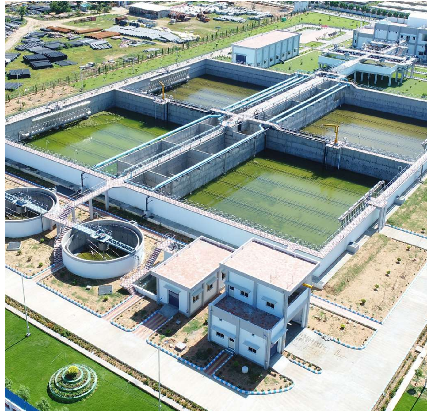
55 MLD Wastewater Treatment Plant, Nellore, Andhra Pradesh
