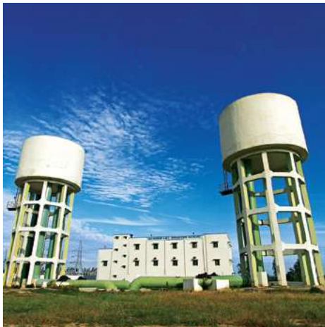
Ali Sagar Lift Irrigation Scheme, Telangana
