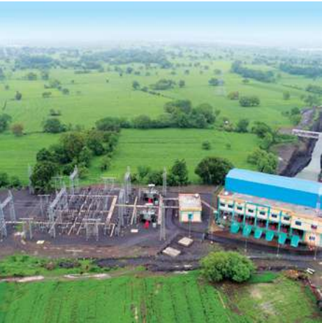
Mohanpura Lift Irrigation Project, Madhya Pradesh
