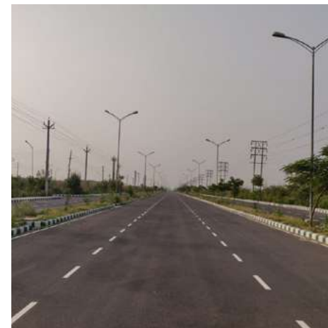
Integrated infrastructure development, Rohtak, Haryana
