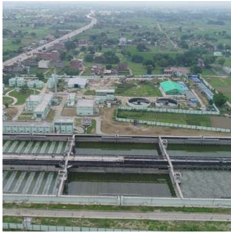
120 MLD Wastewater Treatment Plant, Varanasi, Uttar Pradesh
