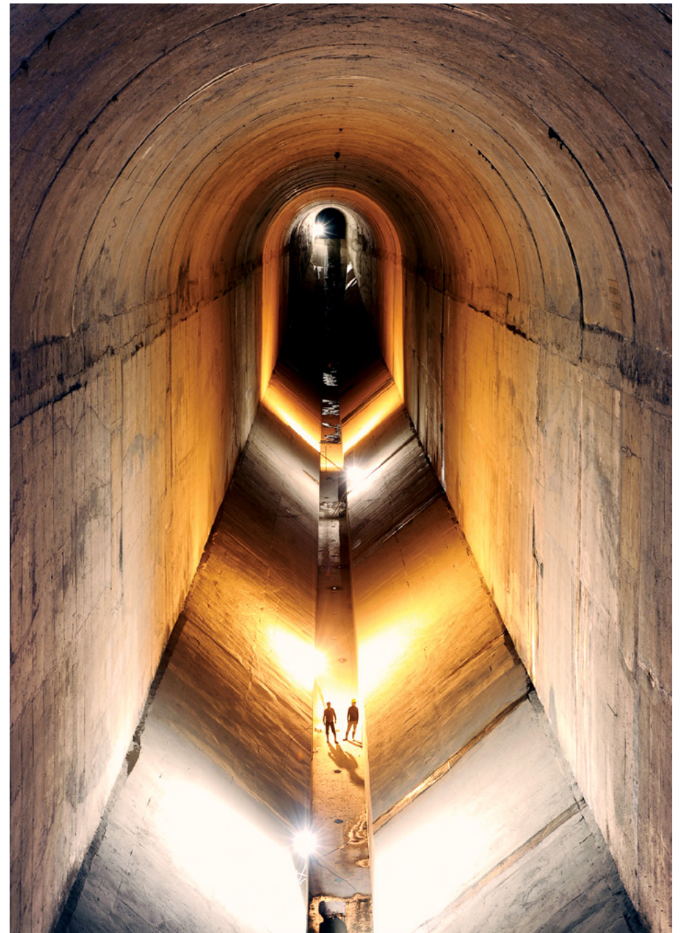
Underground desilting chamber, Parbati
