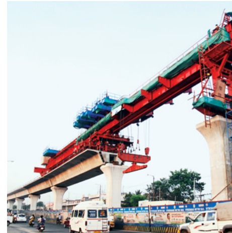
Girder erection for Hyderabad Metro
