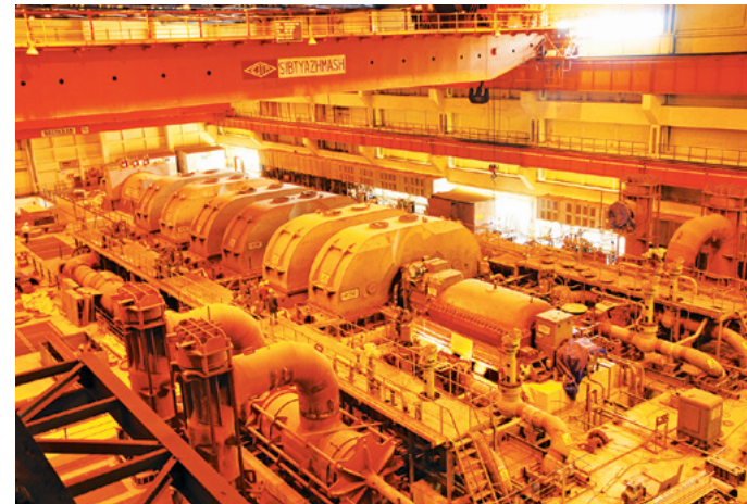
Turbine erection for Kudankulam nuclear power project
