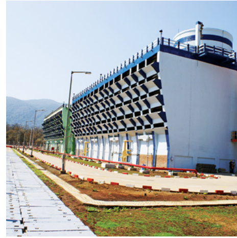
Induced draft cooling tower, Kaiga
