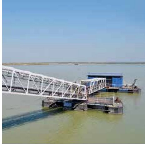
Floating barge intake, Sahibganj, Jharkhand
