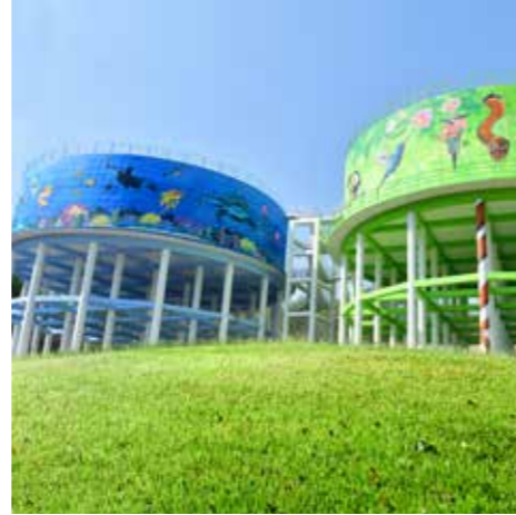
Elevated Storage Reservoir, Pune, Maharashtra
