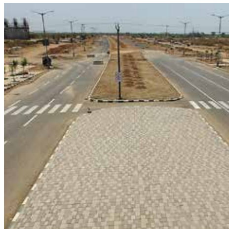
Green-field development at Dholera, Gujarat
