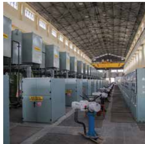
Pump house at Hanamapur, Karnataka
