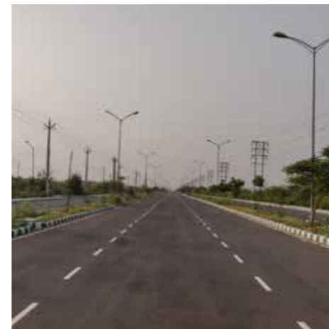
Integrated infrastructure development, Rohtak, Haryana
