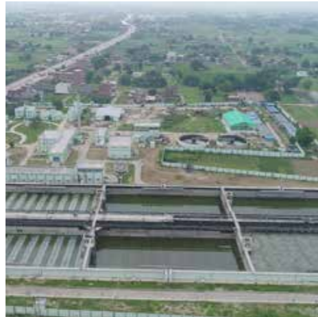
120 MLD Wastewater Treatment Plant, Varanasi, Uttar Pradesh
