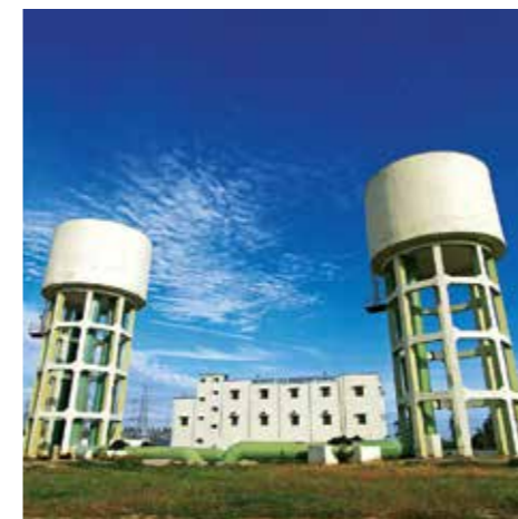
Ali Sagar Lift Irrigation Scheme, Telangana
