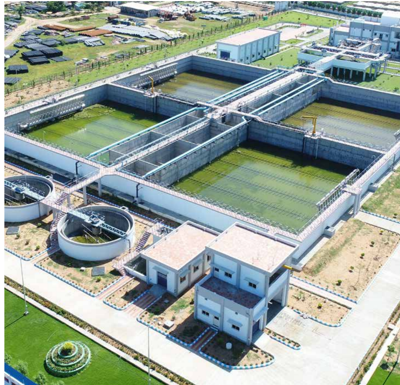
55 MLD Wastewater Treatment Plant, Nellore, Andhra Pradesh
