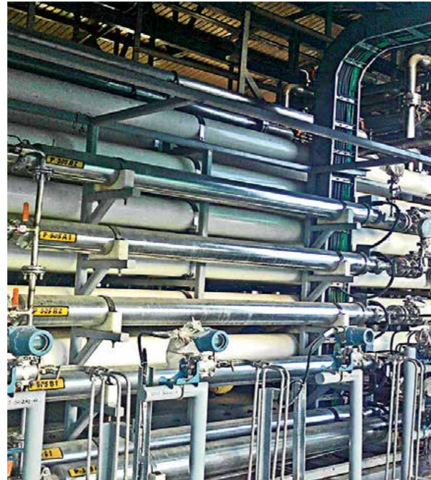
Reverse osmosis technology at a desalination project
