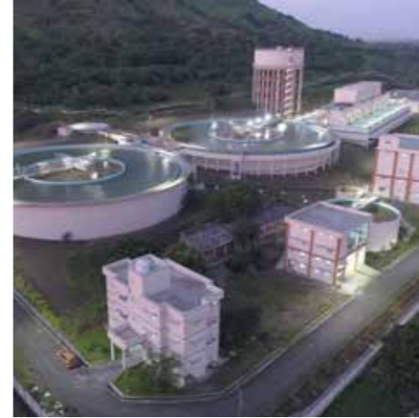
137 MLD Water Treatment Plant at Nashik, Maharashtra
