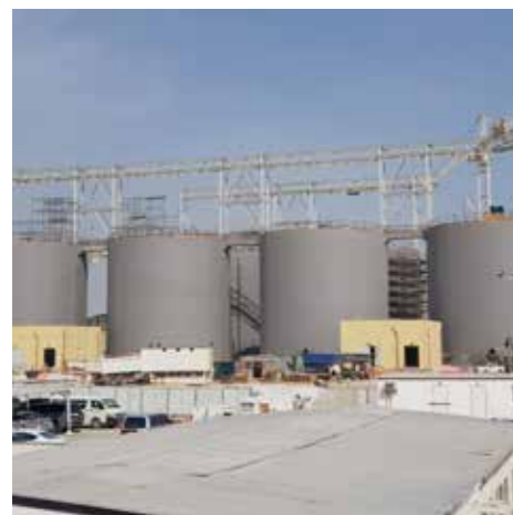
Anaerobic digesters
