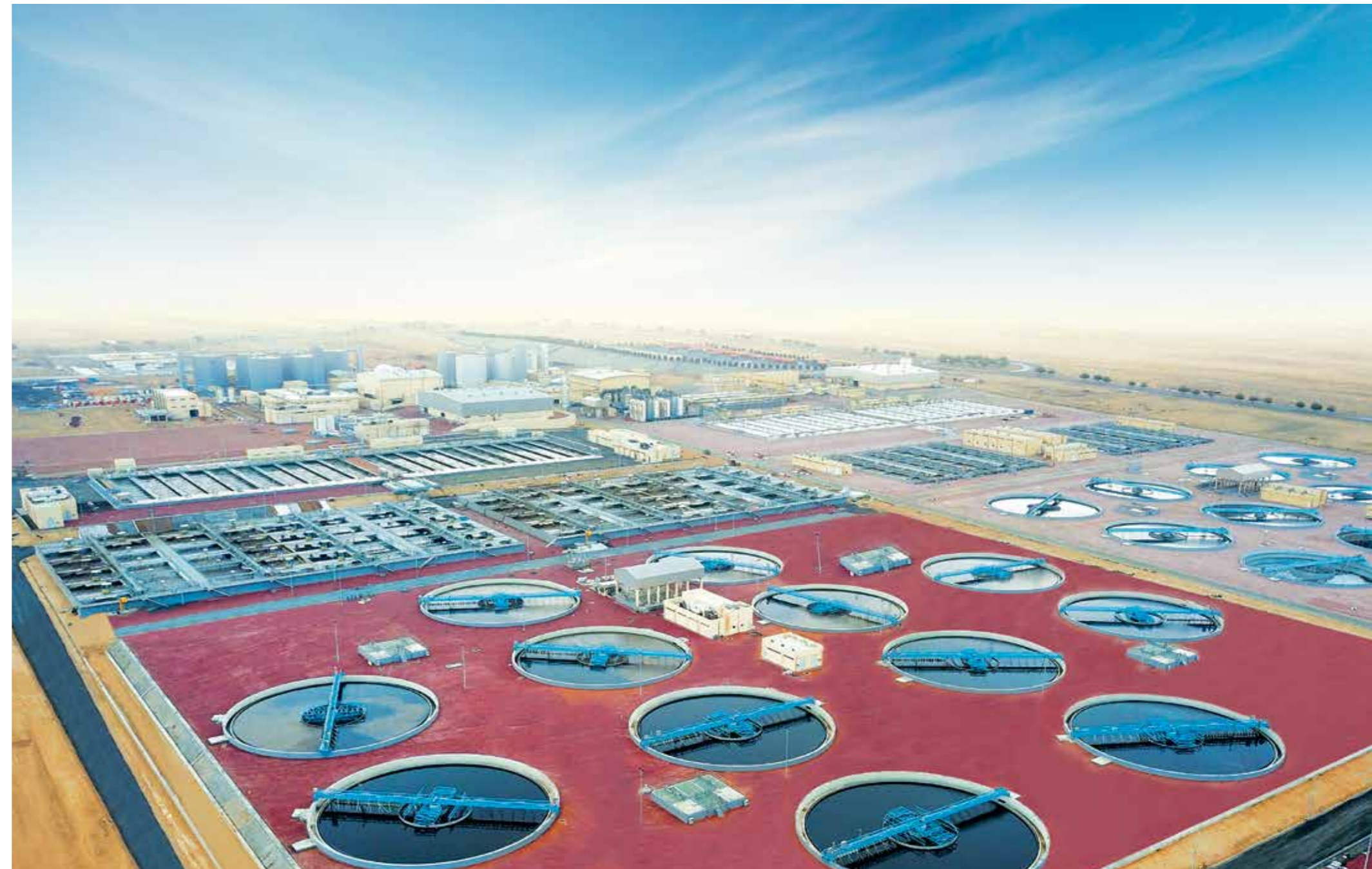
375 MLD Wastewater Treatment Plant, Jebel Ali, UAE
