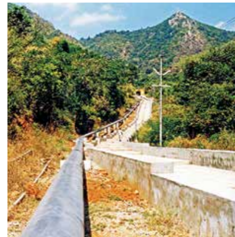
Pipeline installed on steep gradients
