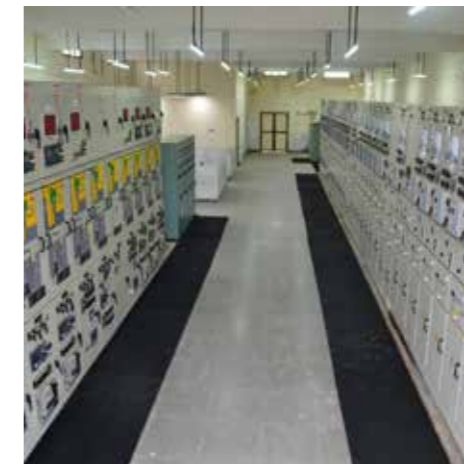
Substation, Bidkin, Maharashtra
