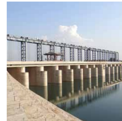
Kharkai Barrage, Jharkhand
