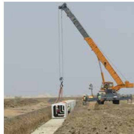
Precast duct laying at Amaravati, Andhra Pradesh
