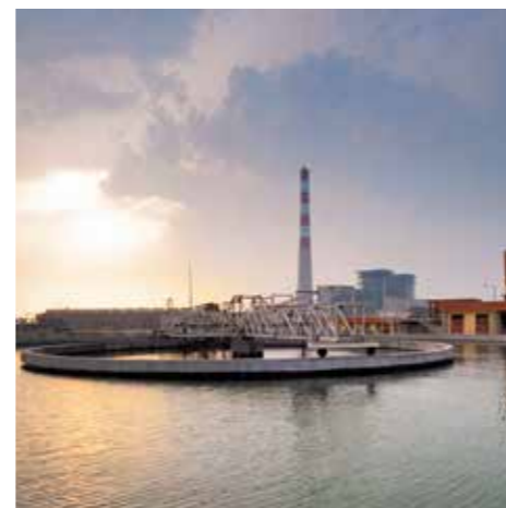
Plant Water System, Sagardighi, West Bengal
