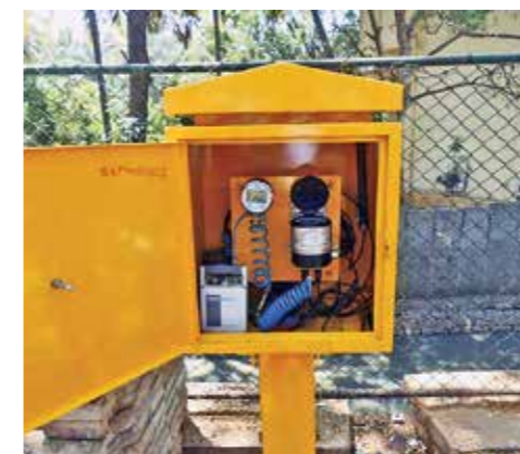
District meter cabinet
