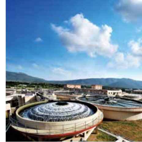
181 MLD Water Treatment Plant, Vellore, Tamil Nadu
