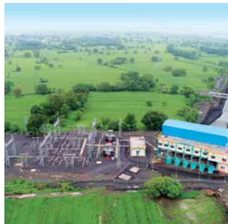
Mohanpura Lift Irrigation Project, Madhya Pradesh
