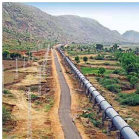
Transmission Mains, Bisalpur, Rajasthan
