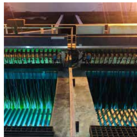
UV Disinfection System
