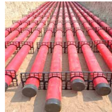
PLB Duct at Amaravati, Andhra Pradesh
