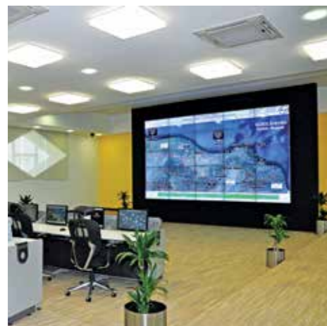
Real-time Project monitoring with SCADA
