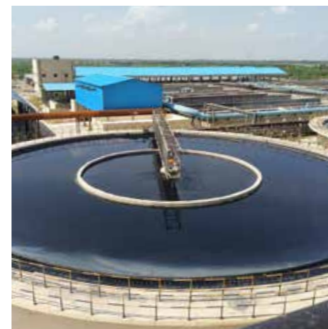
100 MLD Common Effluent Treatment Plant, Narol, Gujarat
