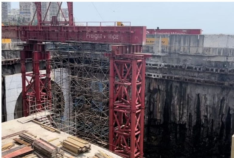
The point where the breakthrough of the second tunnel is expected | Manasi Phadke, ThePrint
