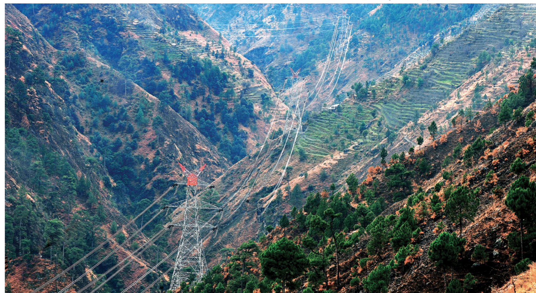
400 kV double circuit Karcham Wangtoo–Abdullapuri transmission line
