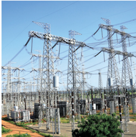
765 kV ultra high voltage AIS at Unnao
