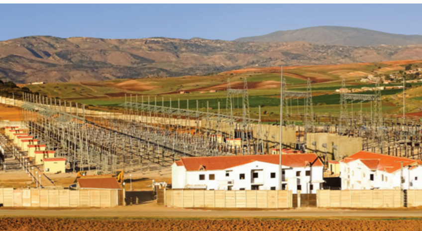
400 kV AIS at Chlef in Algeria
