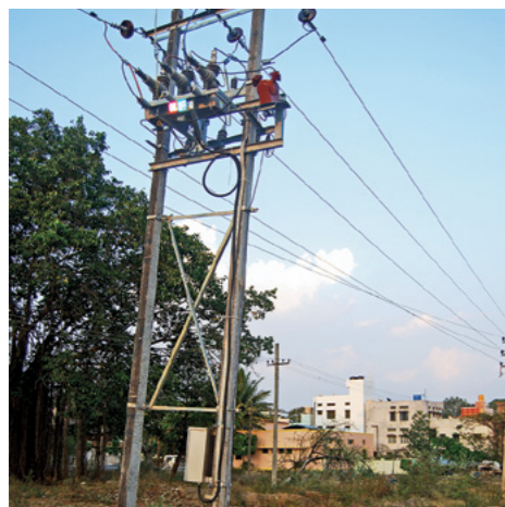
Auto recloser and sectionaliser works
