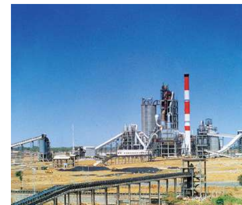
Hirmi cement plant, Raipur
