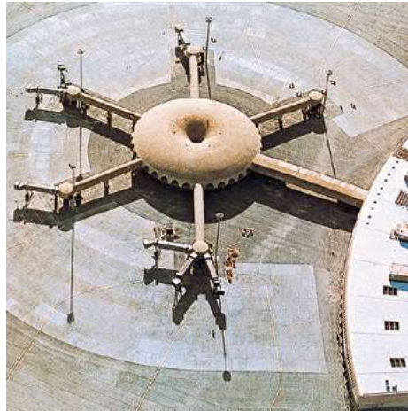
Abu Dhabi International Airport
