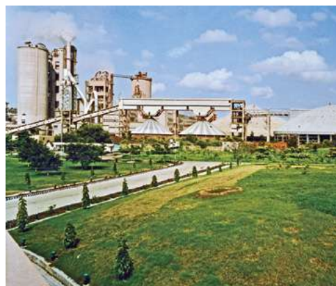
Cement plant at Awarpur, Maharashtra
