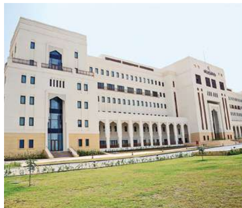
Ministry of Manpower building, Oman
