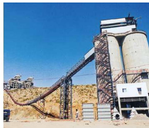
Silos and conveyor at Tadipatri cement plant
