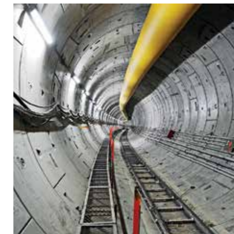
Underground section of Chennai Metro
