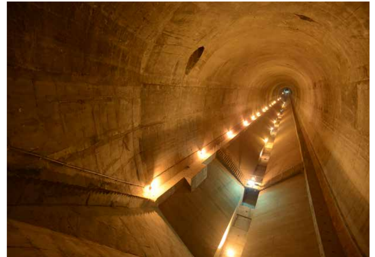
Desilting Chamber, Punatsangchhu
