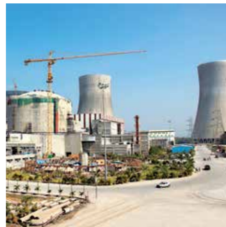
Kakrapar Atomic Power Plant
