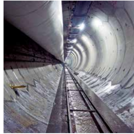
Head Race Tunnel, Tapovan Vishnugad
