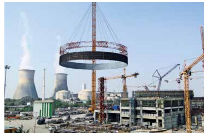
Ring girder erection at Kakrapar Nuclear Power Plant
