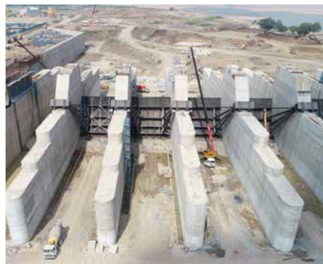
Medigada Gate Erection
