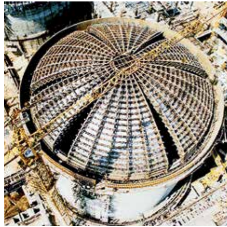
Kaiga atomic power plant
