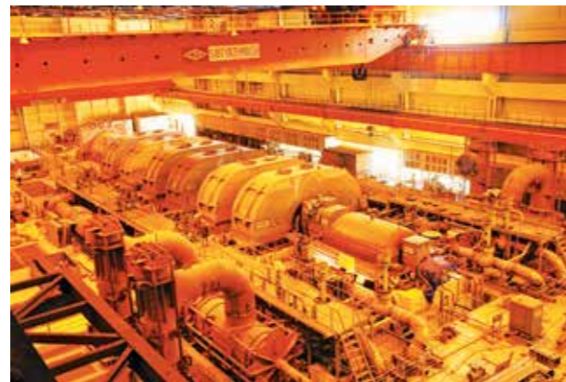
Turbine erection for Kudankulam nuclear power project
