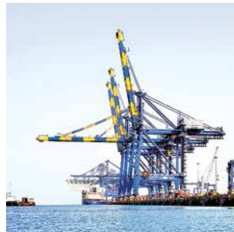
Container terminal at Mundra, Gujarat
