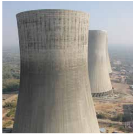
Kakrapar Atomic Power Plant
