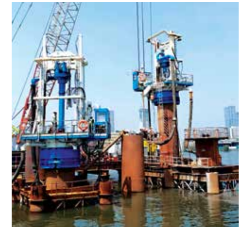
Reverse Circulation Drilling (RCD) rigs in operation at MTHL, Mumbai
