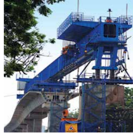
Girder erection for Chennai Metro
