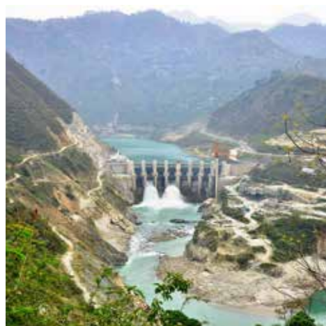
Earthen dam, Chhattisgarh
