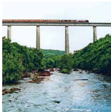
Panvel Nadi viaduct
