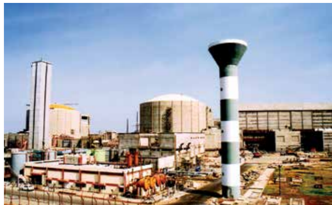
Tarapur atomic power plant
