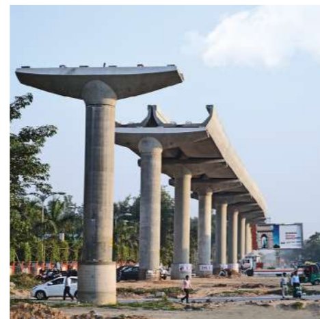
Precast 'U' girder for Delhi Metro
