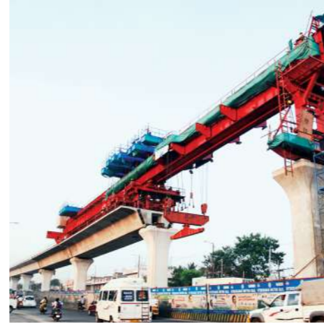
Girder erection for Hyderabad Metro
