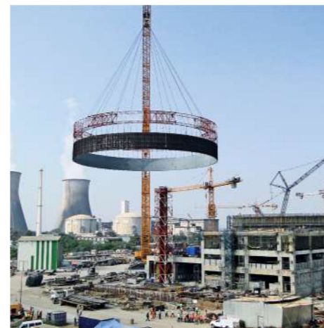
Ring girder erection at Kakrapar Nuclear Power Plant
