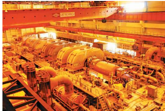
Turbine erection for Kudankulam nuclear power project
