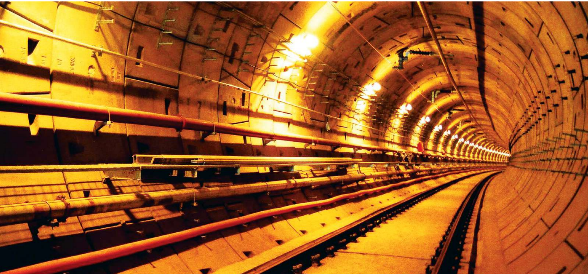
Underground section of Delhi Metro
