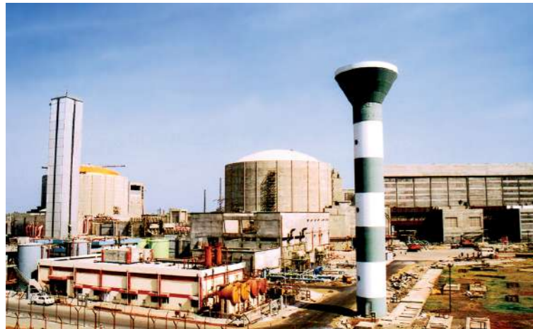
Tarapur atomic power plant
