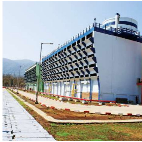
Induced draft cooling tower, Kaiga
