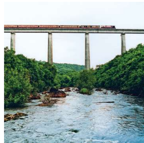
Panvel Nadi viaduct
