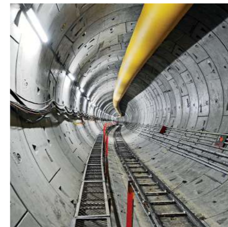
Underground section of Chennai Metro
