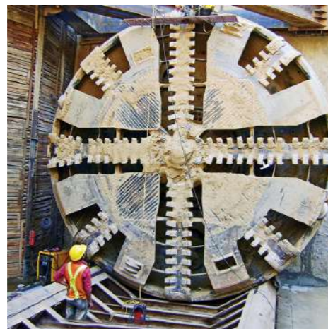
Tunnel Boring Machine
