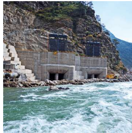
Intake structure at Punatsangchhu, Bhutan
