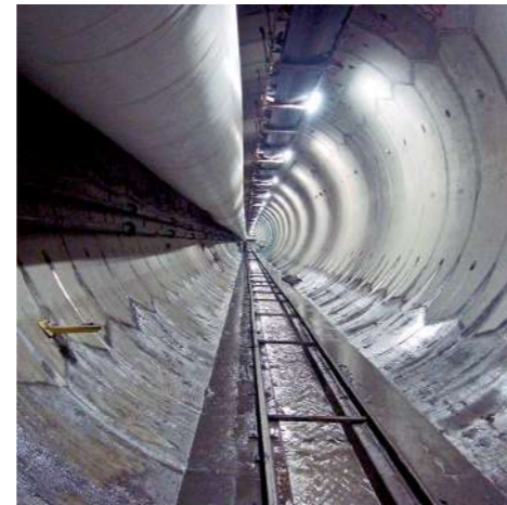
Head Race Tunnel, Tapovan Vishnugad
