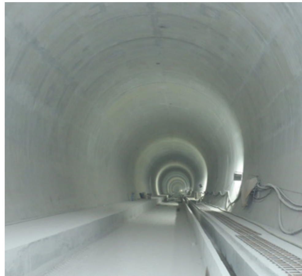
12.9km (6.2km+ 6.7 km) of NATM tunnel in Pkg2 of Rishikesh Karnprayag Railway Line. L&T holds the record of 1012m of NATM in 26 days amidst varying Himalayan geological formations L&T is also executing 15rkmof TBM as part of Pkg 7
