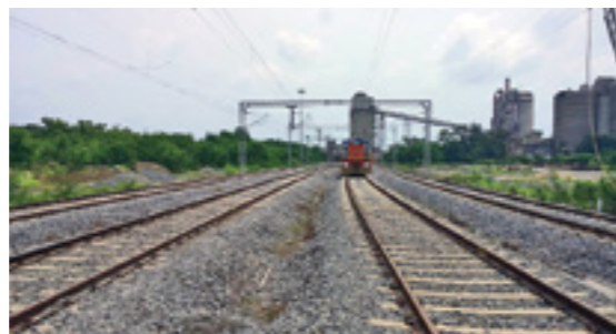
Rail Link to Lafarge Cement Plant, Chattisgarh
