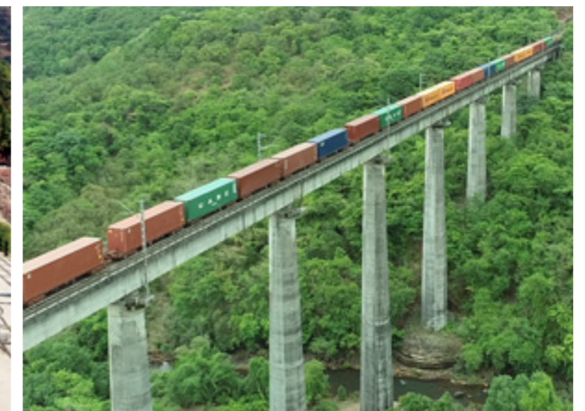
Electrified section of Roha (Mah) - Verna (Goa) of Konkan Railway completed in record time | Majorly single line passing through 70 tunnels and 125 bridges.
