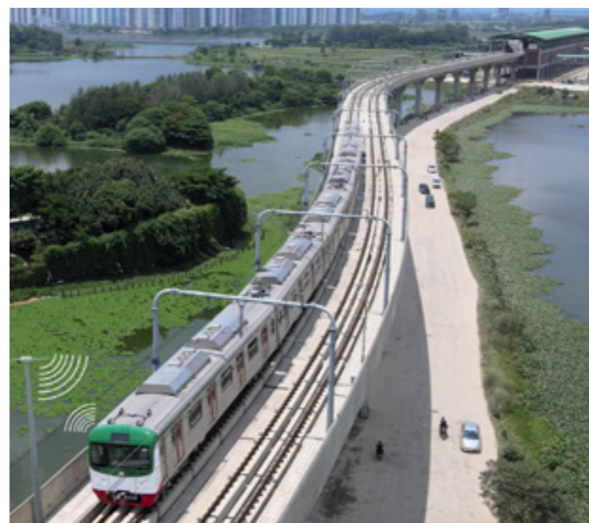
Communication Based Train Control and Signalling
