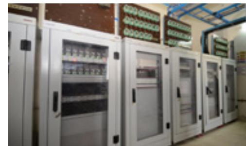
Electronic Interlocking panels
