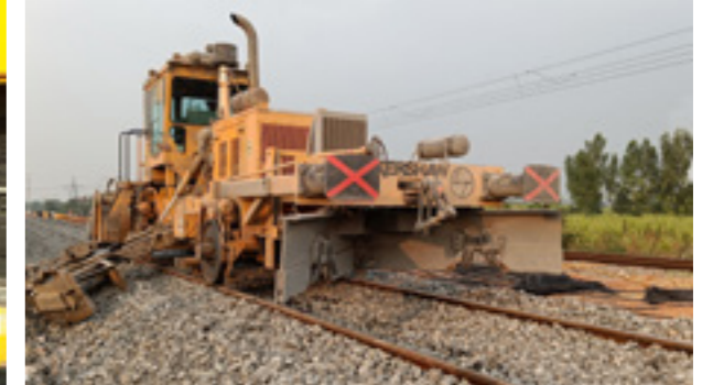
Ballast Profiling (Kershaw)
