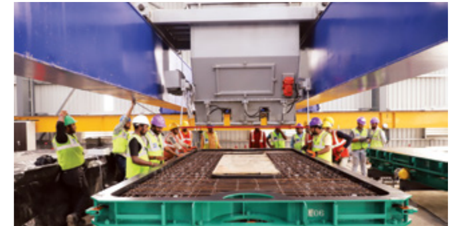
Slab Casting through Automated Concrete Spreader.
