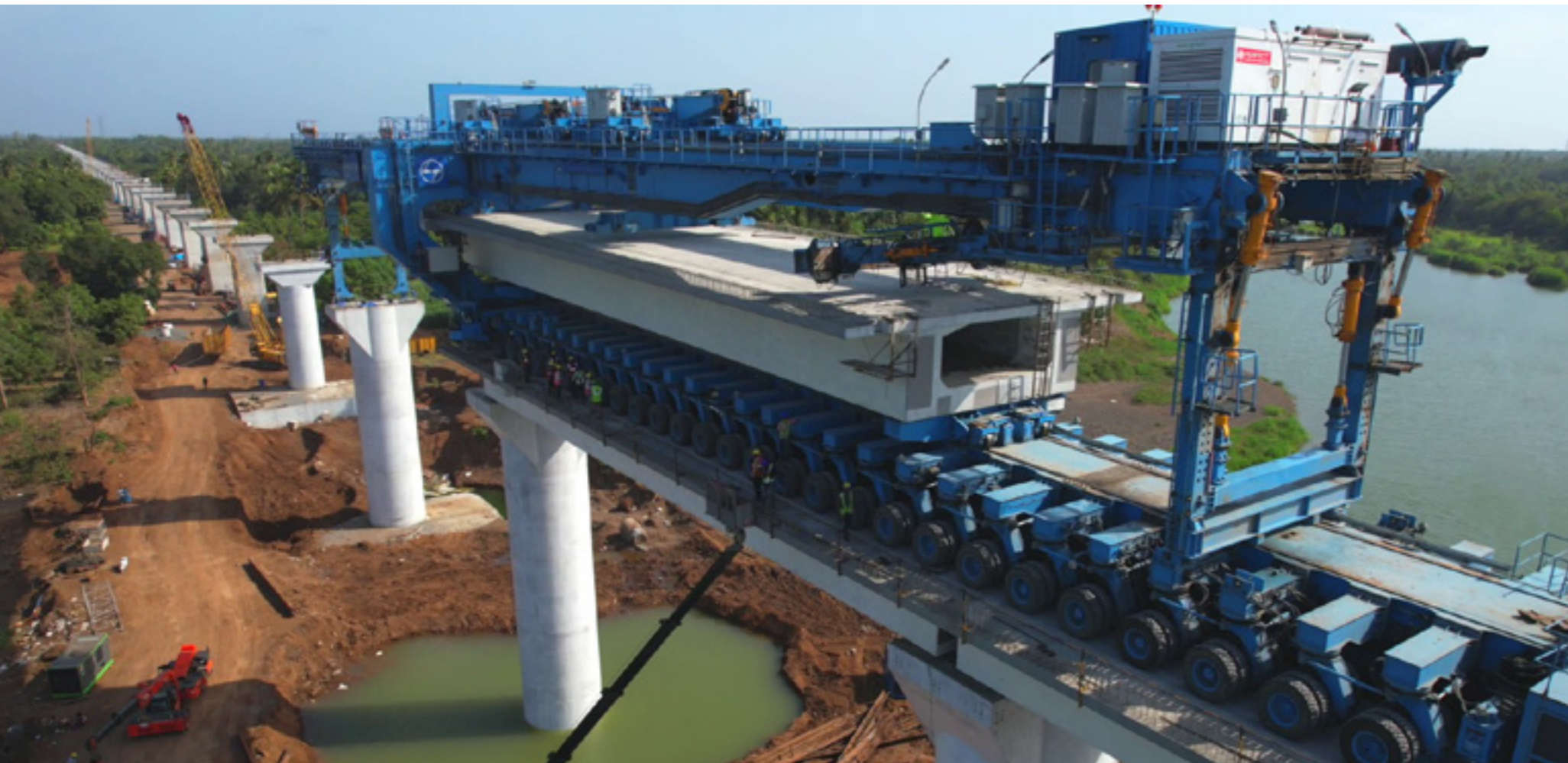
Full Span Launching Gantry & Girder Transporter - MAHSR, India
