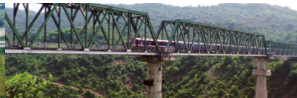
Gambhir khad bridge in Jammu Udhampur Rail link
