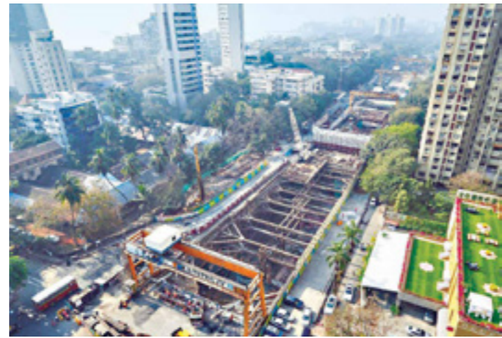
Station at Cuffe Parade - creating infrastructure amidst dense constructed space
