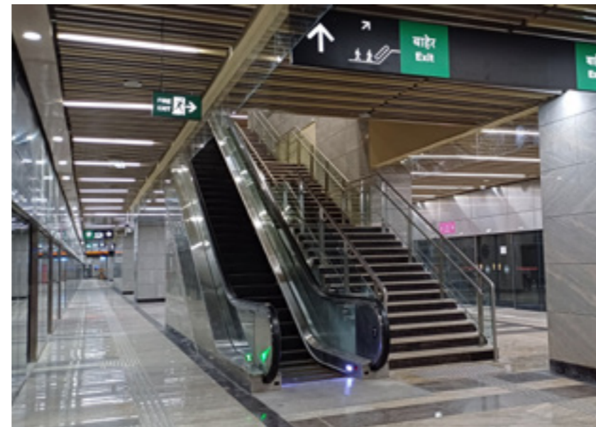
Underground Station Building Mumbai Metro Line 4
