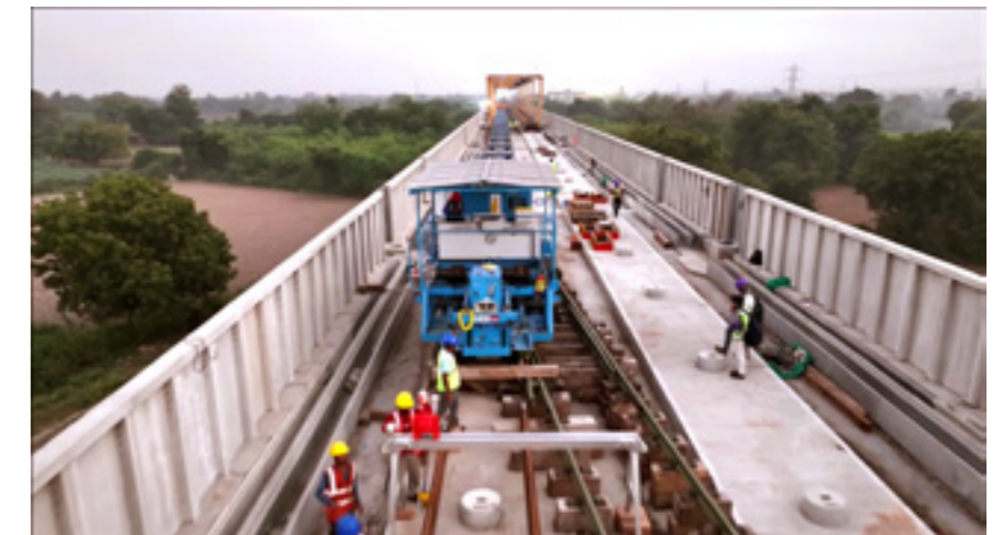
Rail Feeder car
