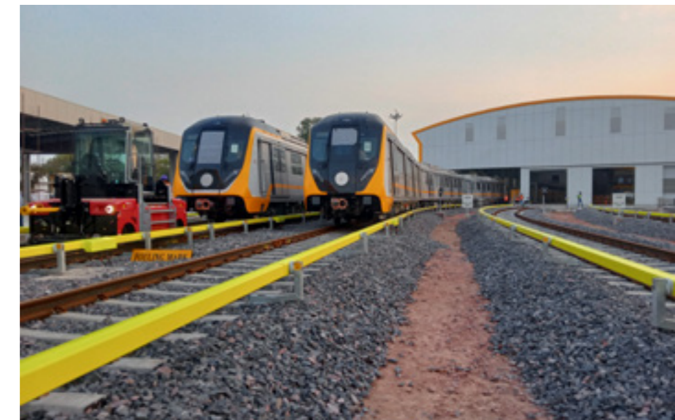
Agra Metro (56tkm) Track & DC Traction with 3rd rail system
