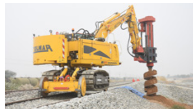
Mechanised Cylindrical Mast foundations in WDFC
