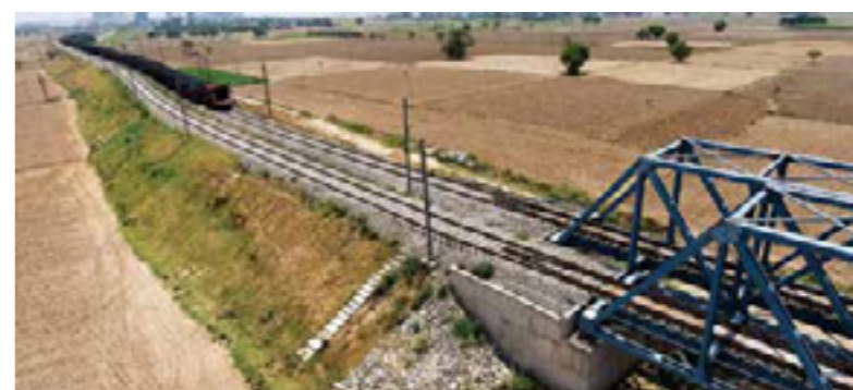
45 km coal link and coal handling facilities - Nabha Power, Punjab
