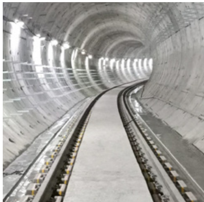
LVT Tracks in Mumbai Metro Line 3
