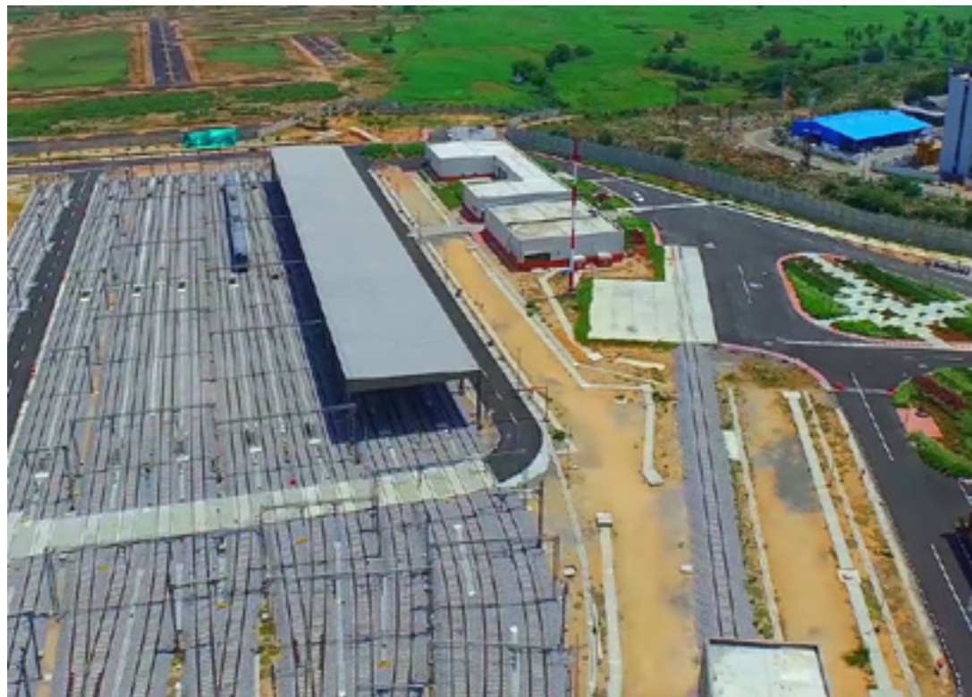
Uppal Depot - Hyderabad Metro
