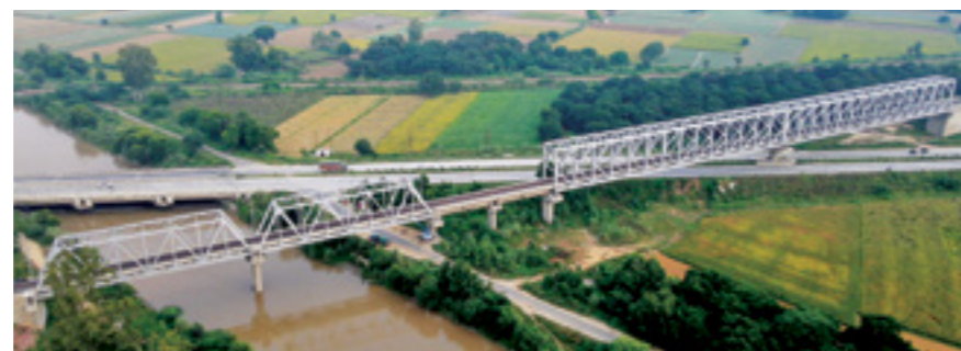
Rail Viaduct crossing Trunk routes - WDFC CP 303
