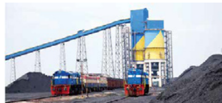
66 km link from mainline to port including bulk material handling for Dhamra port at Odisha.
