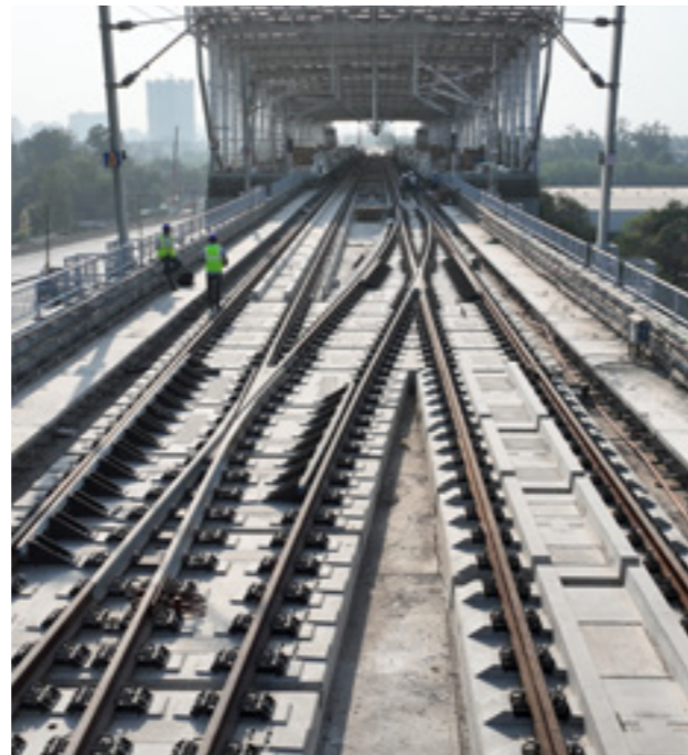
Installed Slab Tracks on Viaduct
