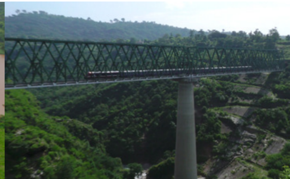
Jhajar khad bridge in Jammu Udhampur Rail link
