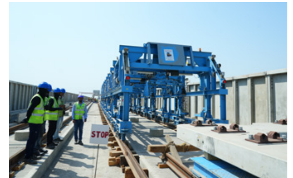
Pre Cast Slab Track Construction in MAHSR Project
