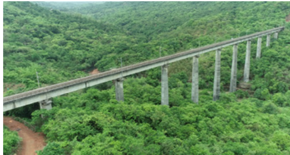
60m high, 420m long Viaduct across Panvel river valley near Ratnagiri India - Built using Incremental launching
