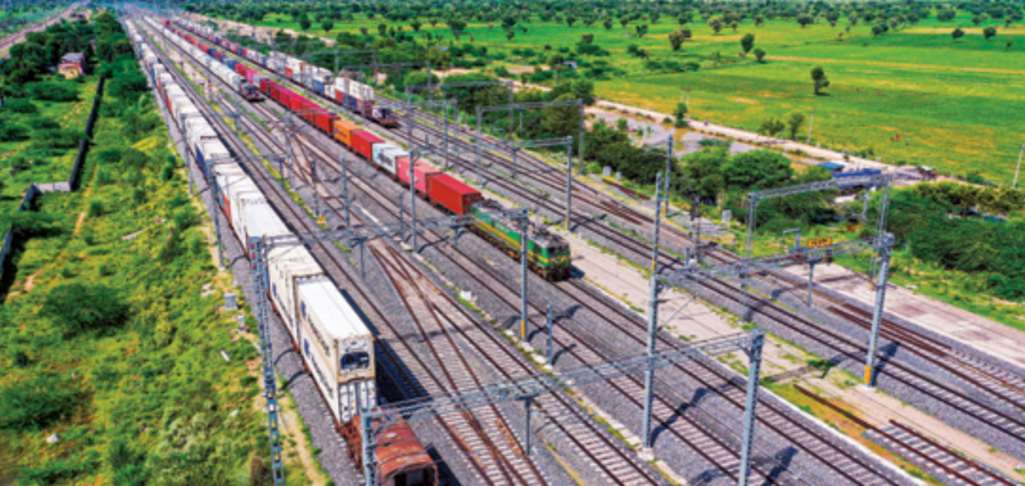
CTP-3R - Iqbalgarh to Vadodara 342 rkm (726 tkm) Commercial Operations started in Priority section - New Phulera Yard
