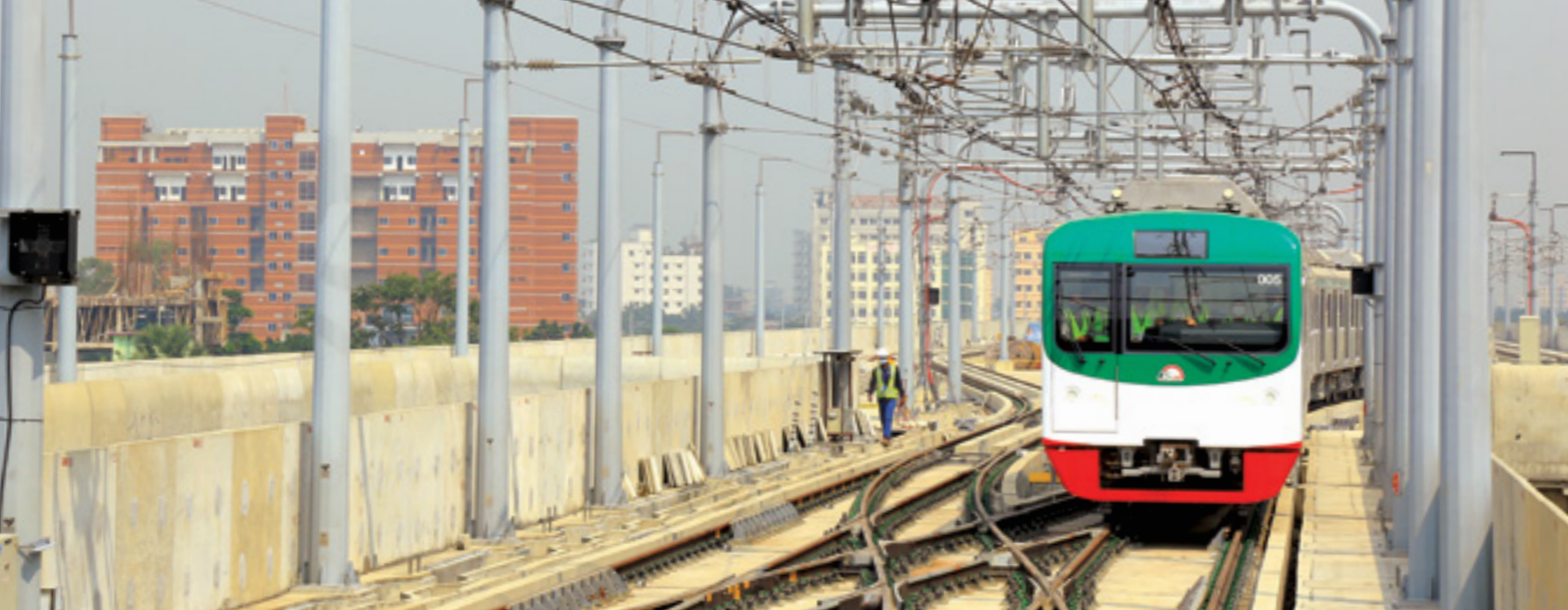
E&M Systems including Overall System Integration
