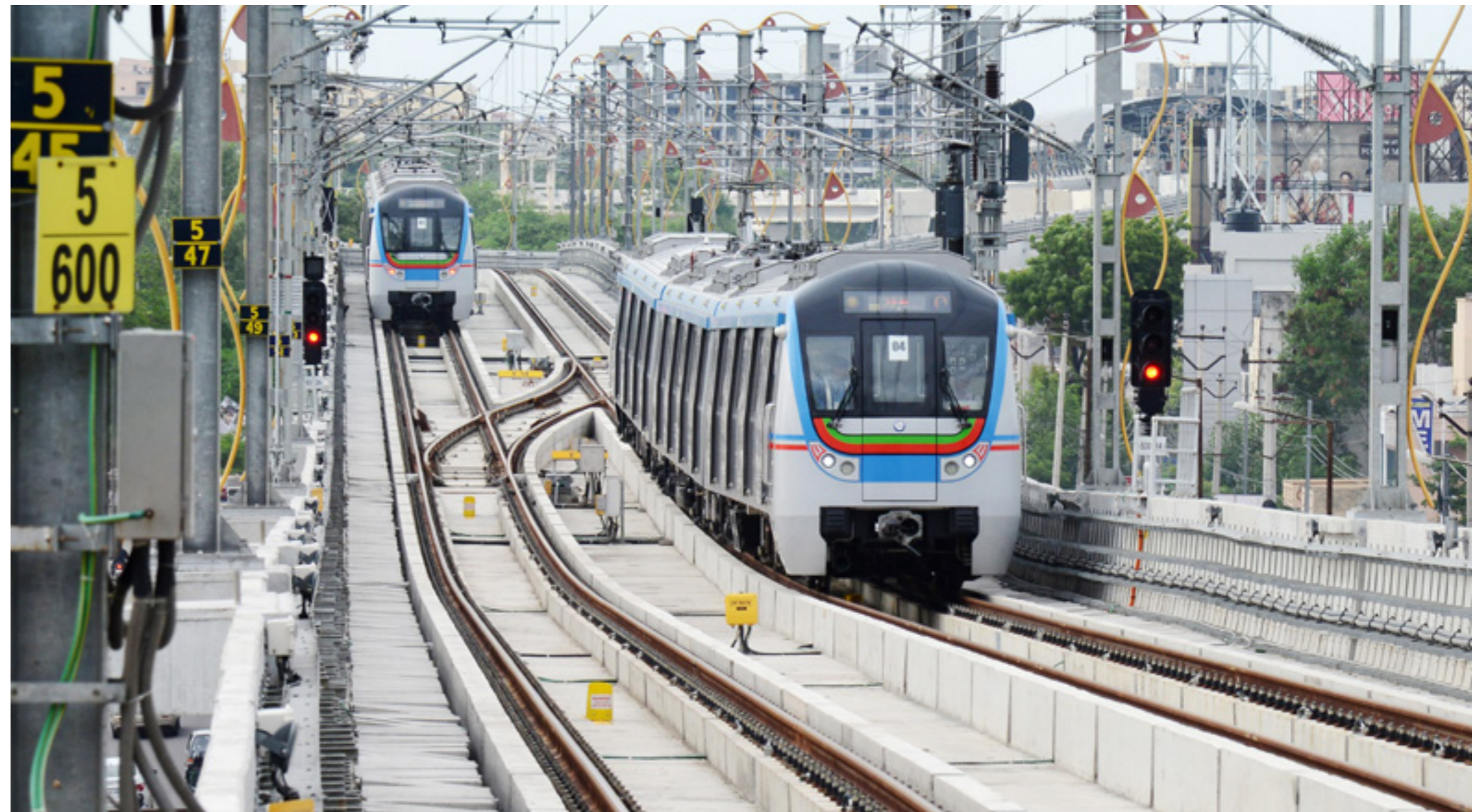
Hyderabad Metro - World's biggest mass transit project on concessionaire basis
