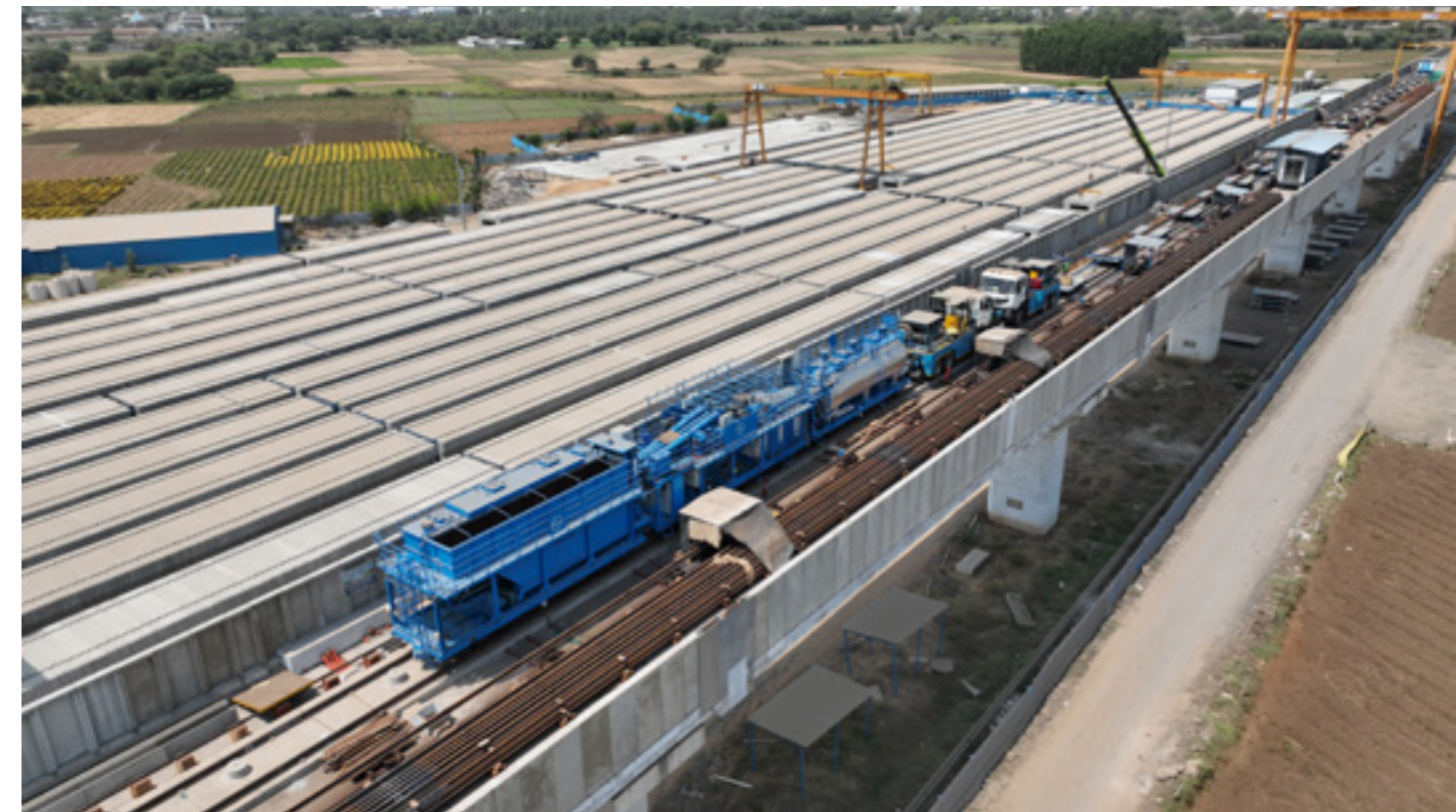
Pre-Cast Slabs in TSMF and Mechanised Track Construction on Viaduct
