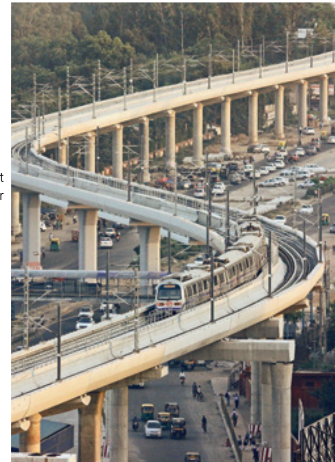
Delhi Metro Phase 3 Delhi - Haryana border - 14.2 km full span U girders.
