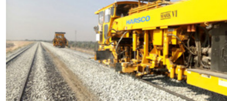
Tamping and Ballast Profiling
