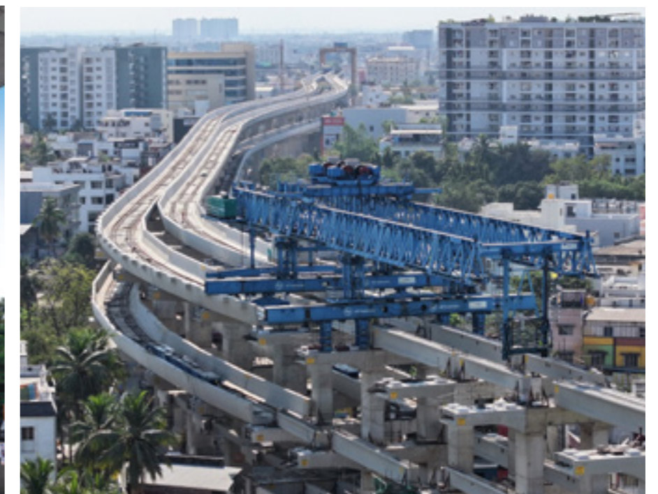
Double Decker Metro Corridor – 3.9 Km – CMRL ECV-01 Project
