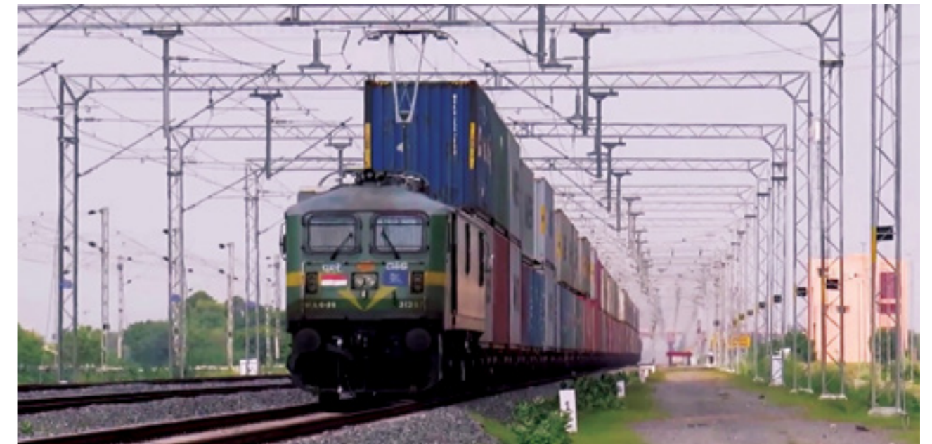
WDFC EMP 4 section - In Regular Commercial Operation
