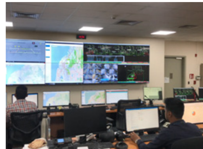
Operations Control Centre
