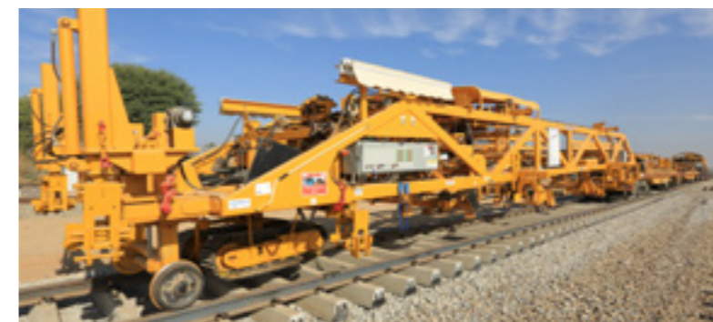
Harsco NTC Machine at WDFC CTP 14 Project
