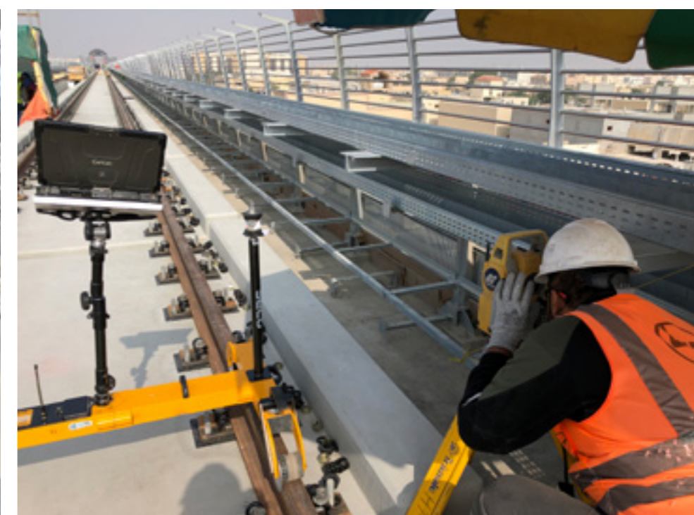
Slab Tracks in Elevated sections of Line 2
