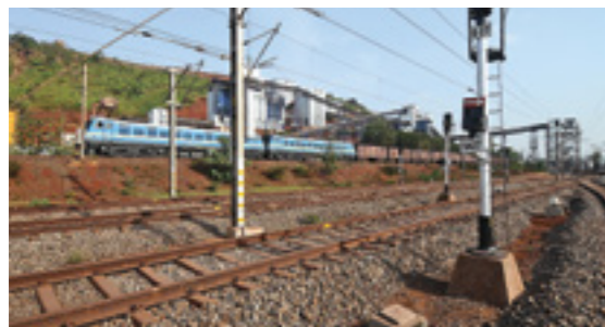
Dedicated Railway Link for Tata Steel, Joda iron ore mines
