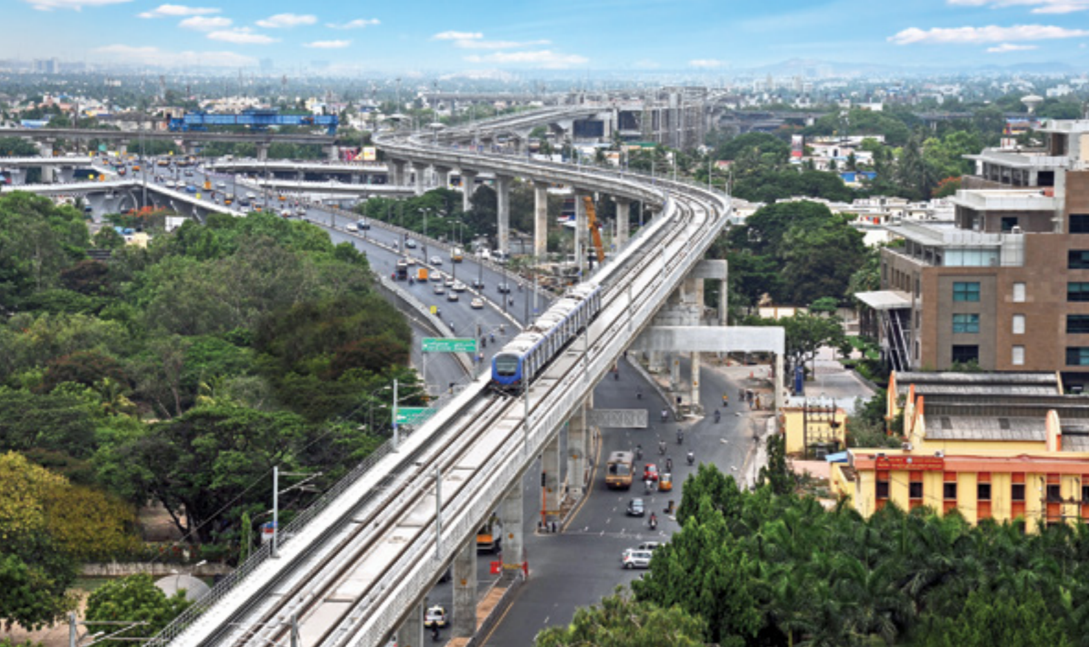
View of the elevated section through one of the many complex alignments
