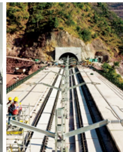
Electrification in Katra-Dharam section using Rigid OCS at major sections
