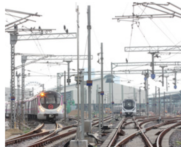
OHE Works at Kalindikunj Depot - Delhi Metro Phase 3
