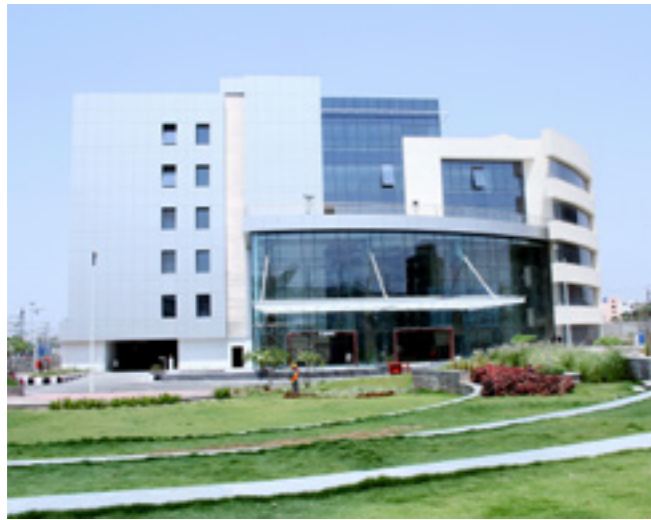
Operation and command centre
