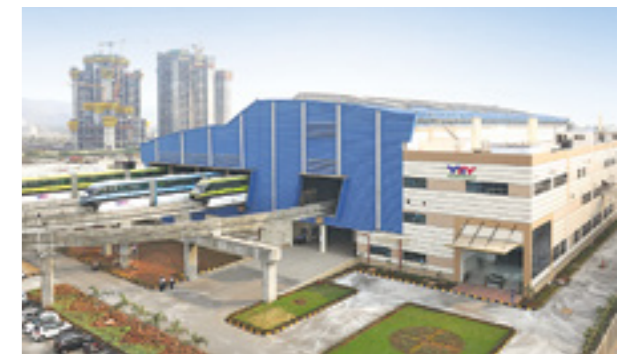
Integrated maintenance depot
