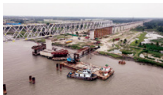
5.13 Km long Rail Bridge over Rupsa River, Bangladesh Railways
