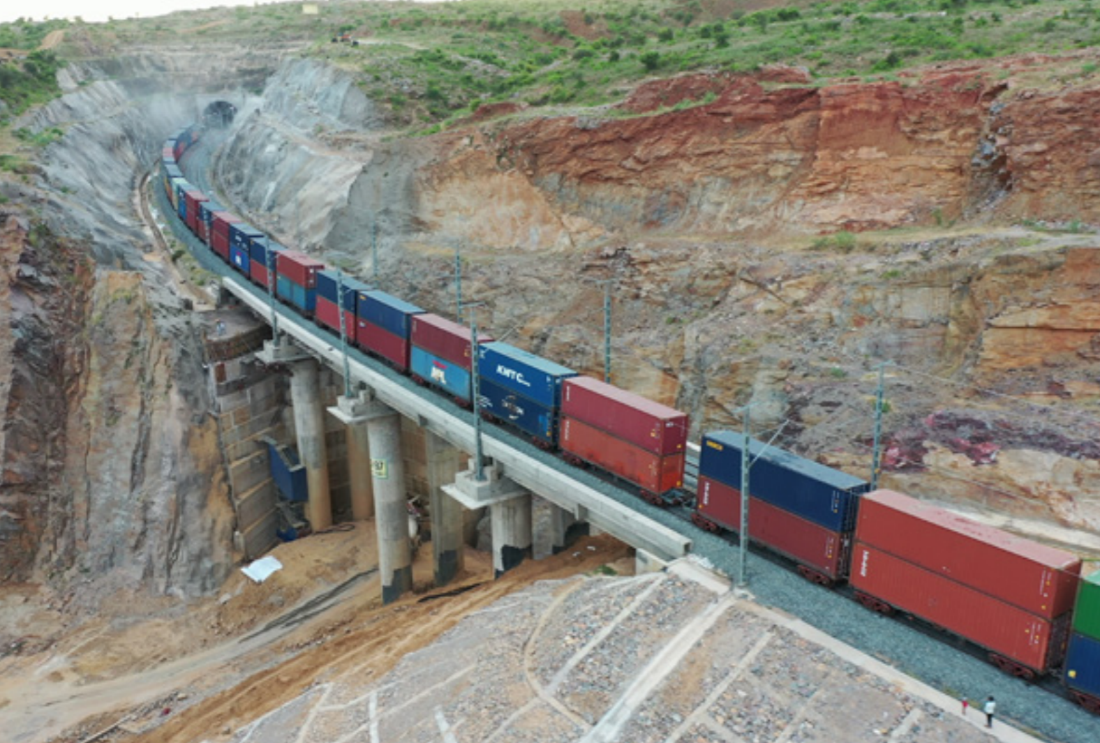
Western Dedicated Freight Corridor, India
