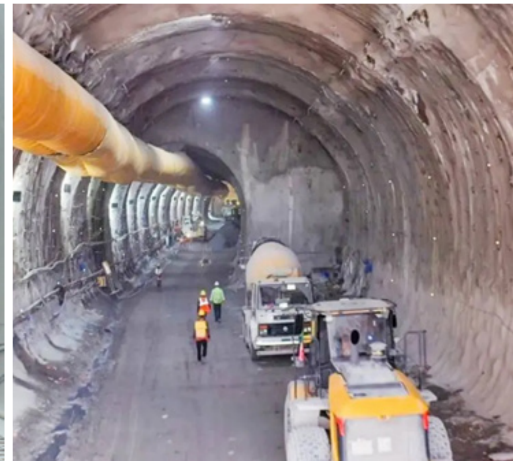
12.9km (6.2km+ 6.7 km) of NATM tunnel in Pkg2 of Rishikesh Karnprayag Railway Line. L&T holds the record of 1012m of NATM in 26 days amidst varying Himalayan geological formations L&T is also executing 15rkmof TBM as part of Pkg 7
