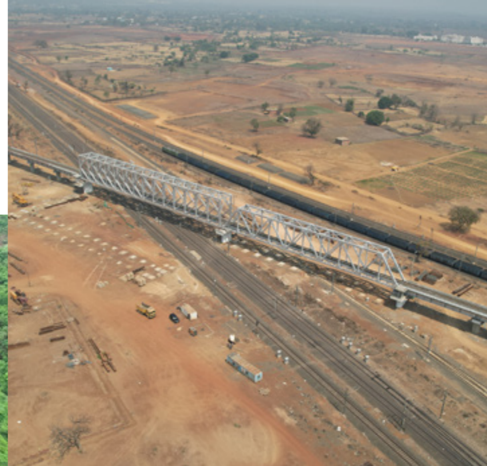
33.4 km Katni Grade Separator
