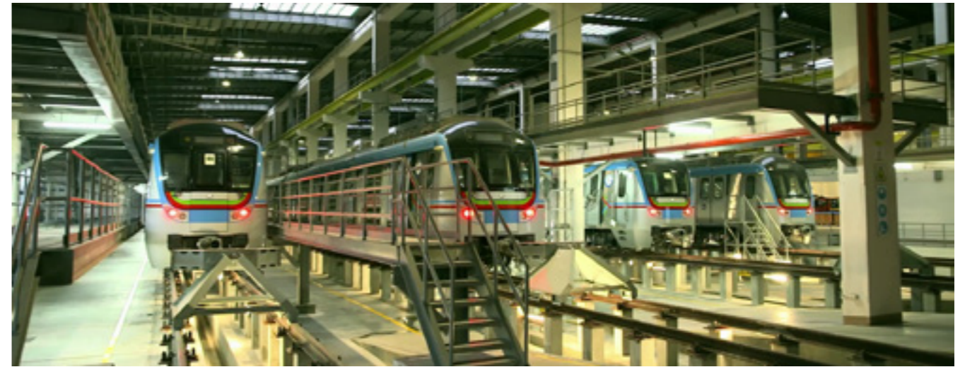
Maintenance Bays in Uppal Depot
