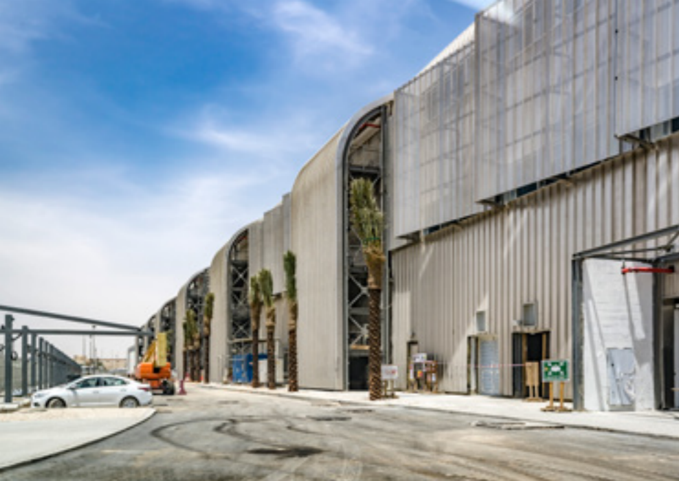
Depot facilities in Riyadh Metro Line 3
