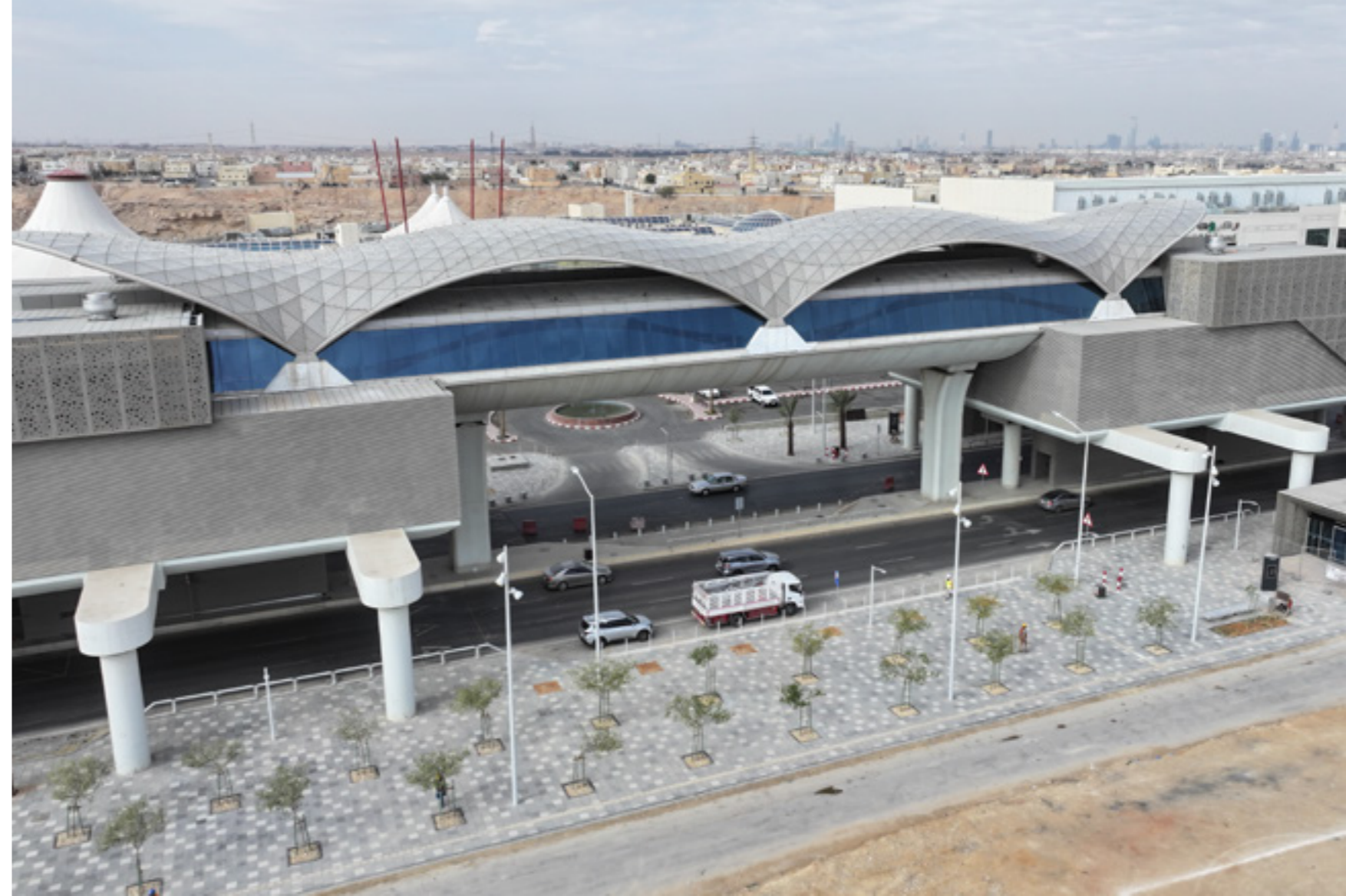
State-of-the-art Station at Riyadh Metro Line 3
