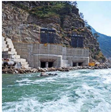
Intake structure at Punatsangchhu, Bhutan
