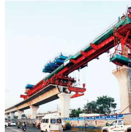
Girder erection for Hyderabad Metro
