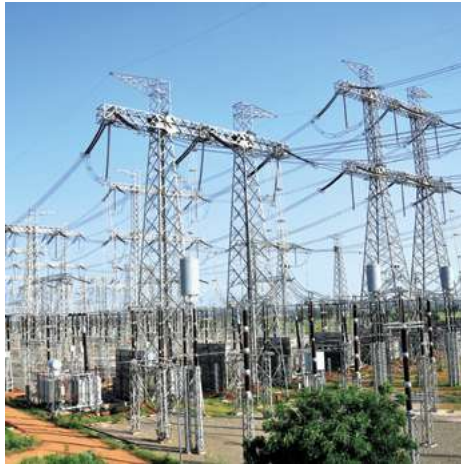
765 kV ultra high voltage AIS at Unnao
