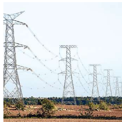
765 kV D/C transmission line at Kudgi
