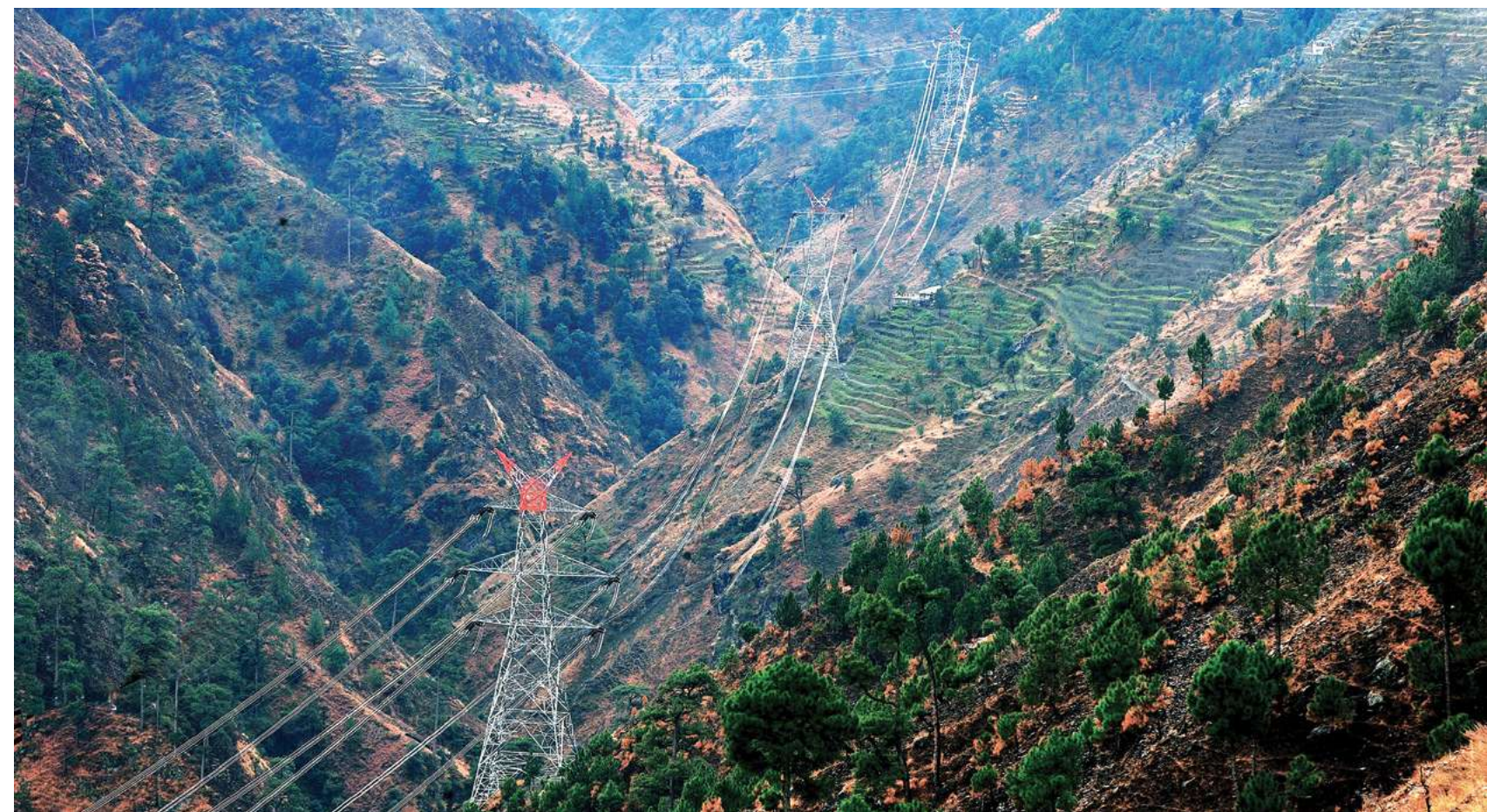
400 kV double circuit Karcham Wangtoo–Abdullapuri transmission line
