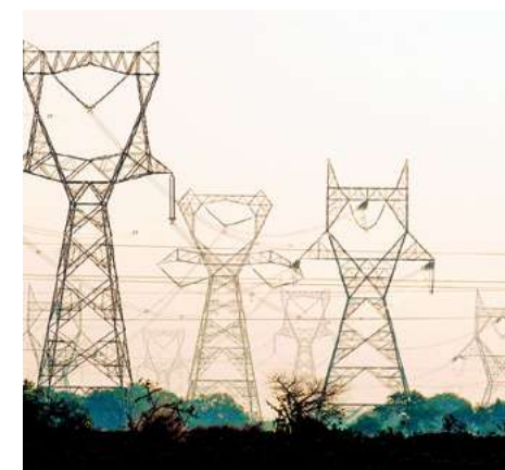
765 kV Sipat-Seoni transmission line
