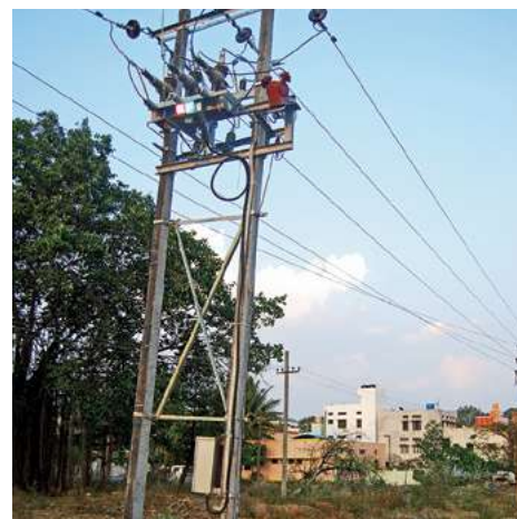
Auto recloser and sectionaliser works
