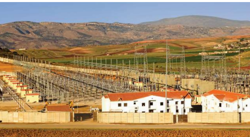
400 kV AIS at Chlef in Algeria
