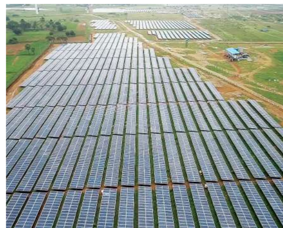
EPC of Solar PV Power Plant
