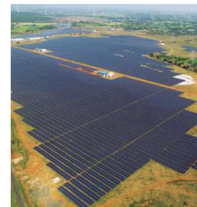
110 MWp Fixed Tilt Solar PV Project in Tamil Nadu
