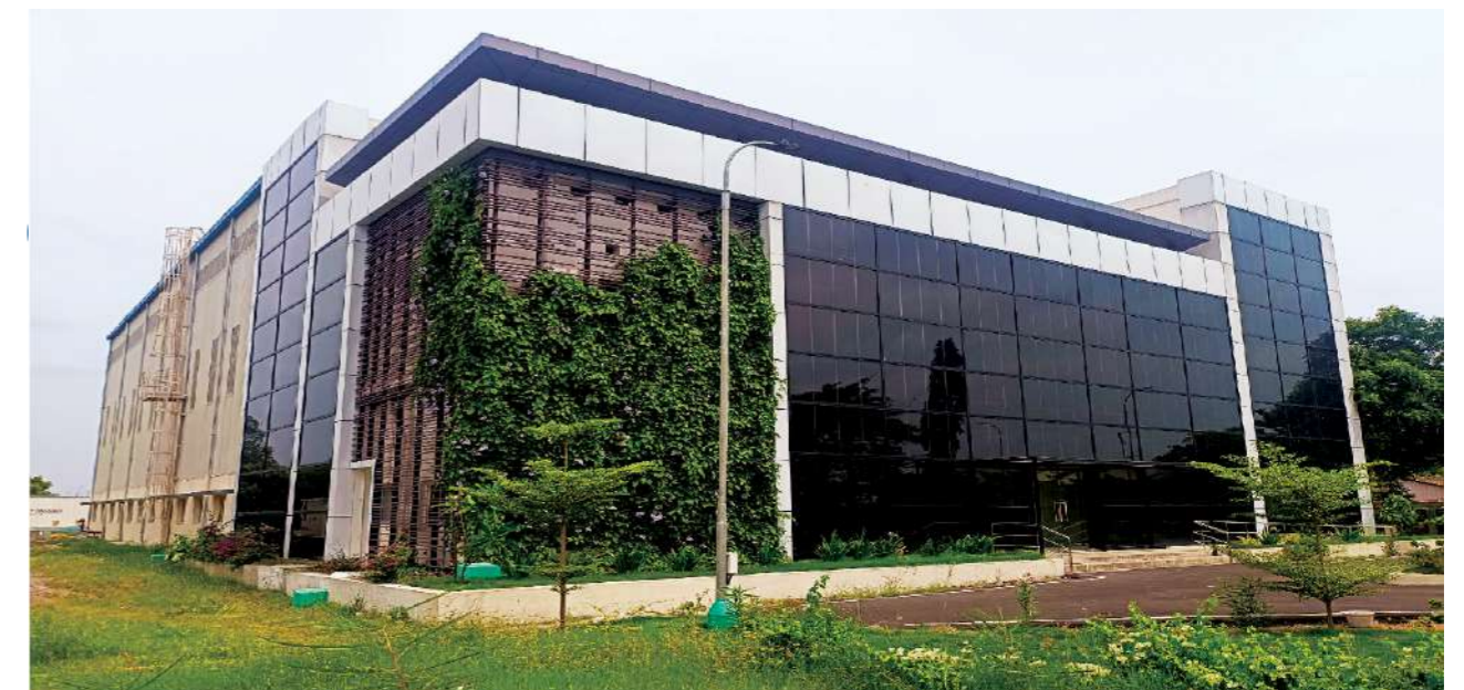
Container Integration Facility - L&T, Kanchipuram
