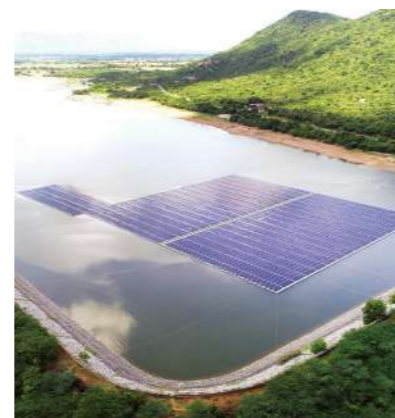
4 MWp Floating Solar PV Project, Tirupati
