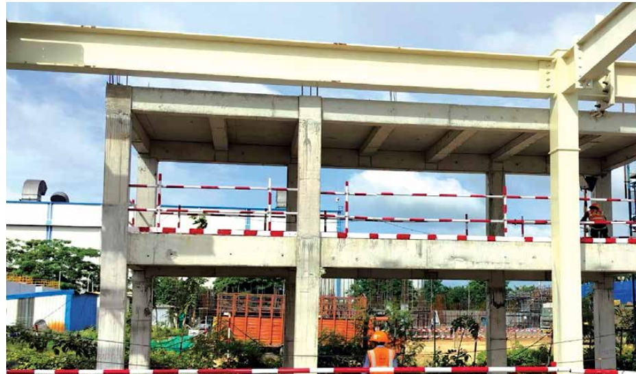
Floor edge barricades installed with toe boards
