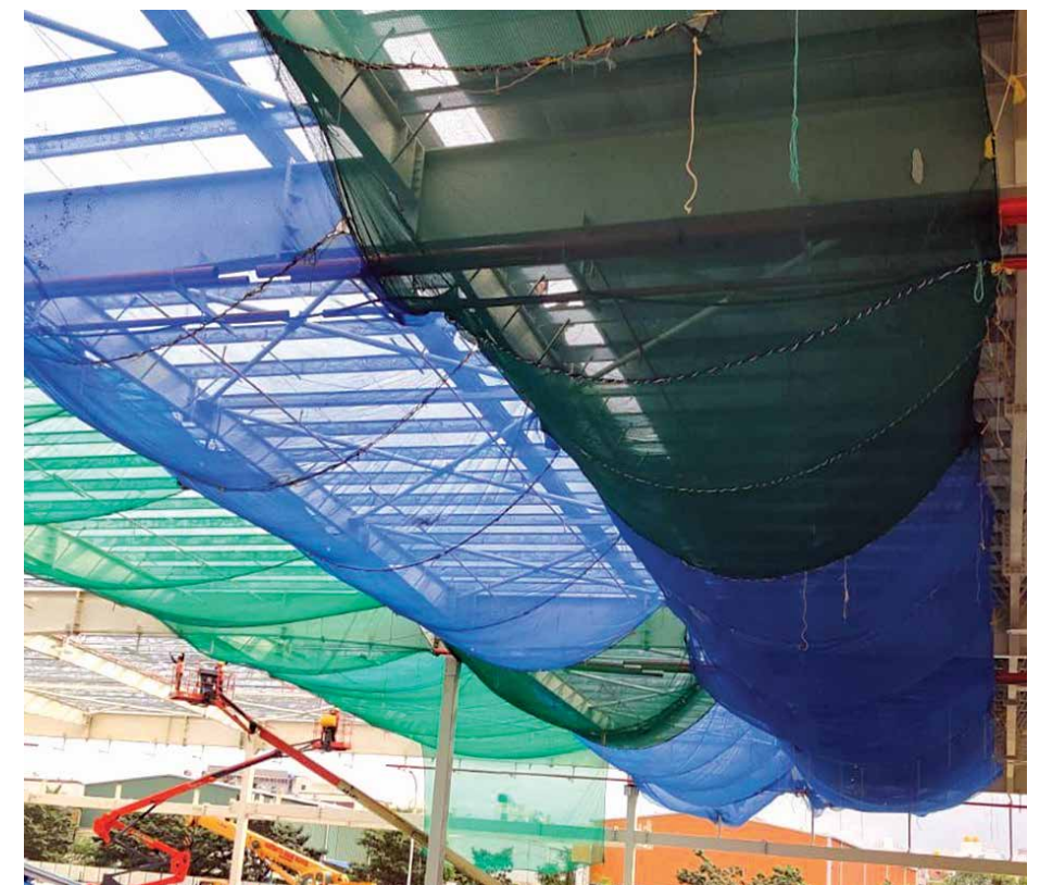
Catch nets installed before the start of roofing
