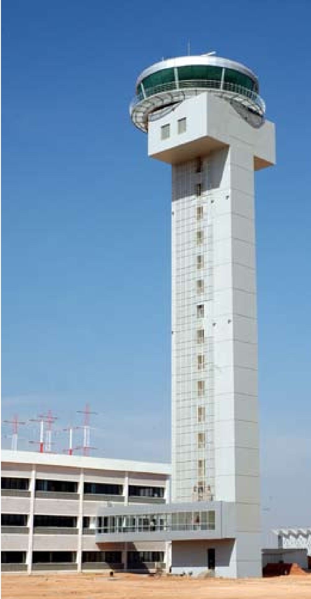
Towering view of the Air Traffic Control Tower
