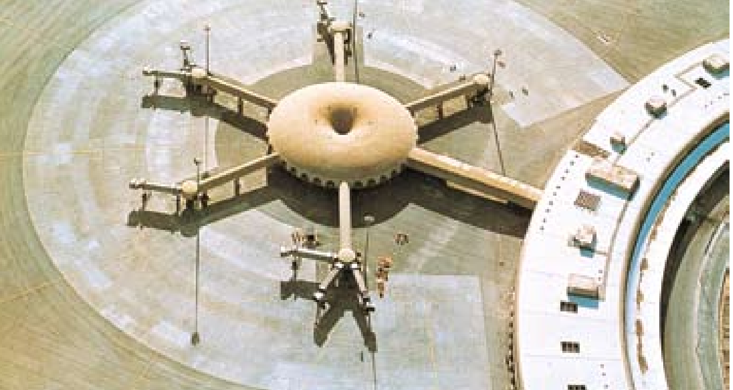
Abu Dhabi International Airport
