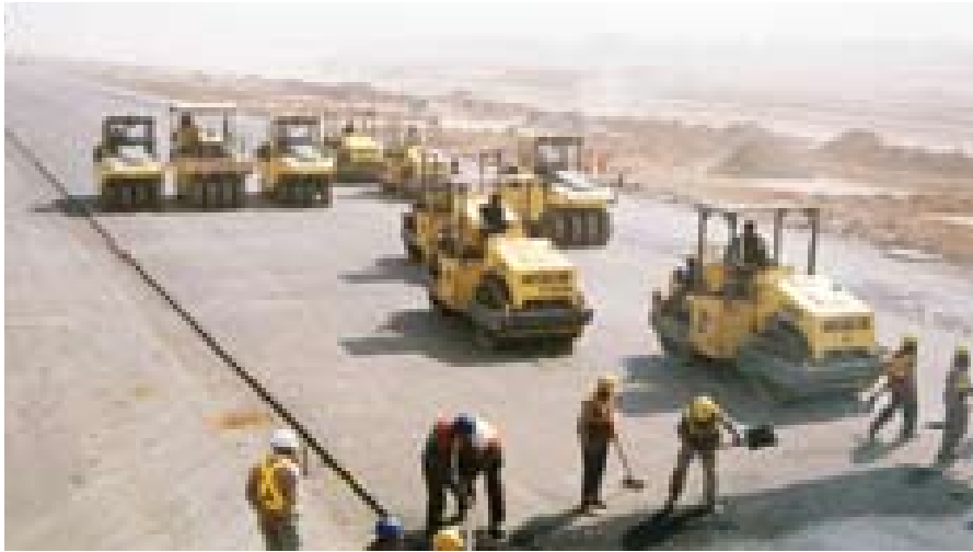
Phase 1A Taxiway Asphaltting works in progress
