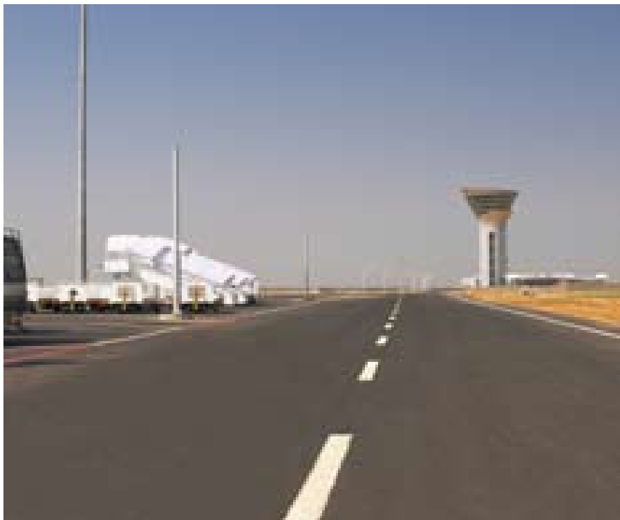
View of ATC & apron service road with lighting masts
