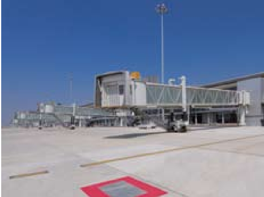
Airside view showing the passenger boarding bridges
