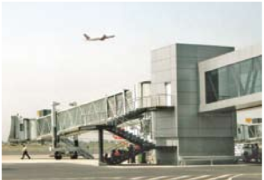
Close up view of a passenger boarding bridge
