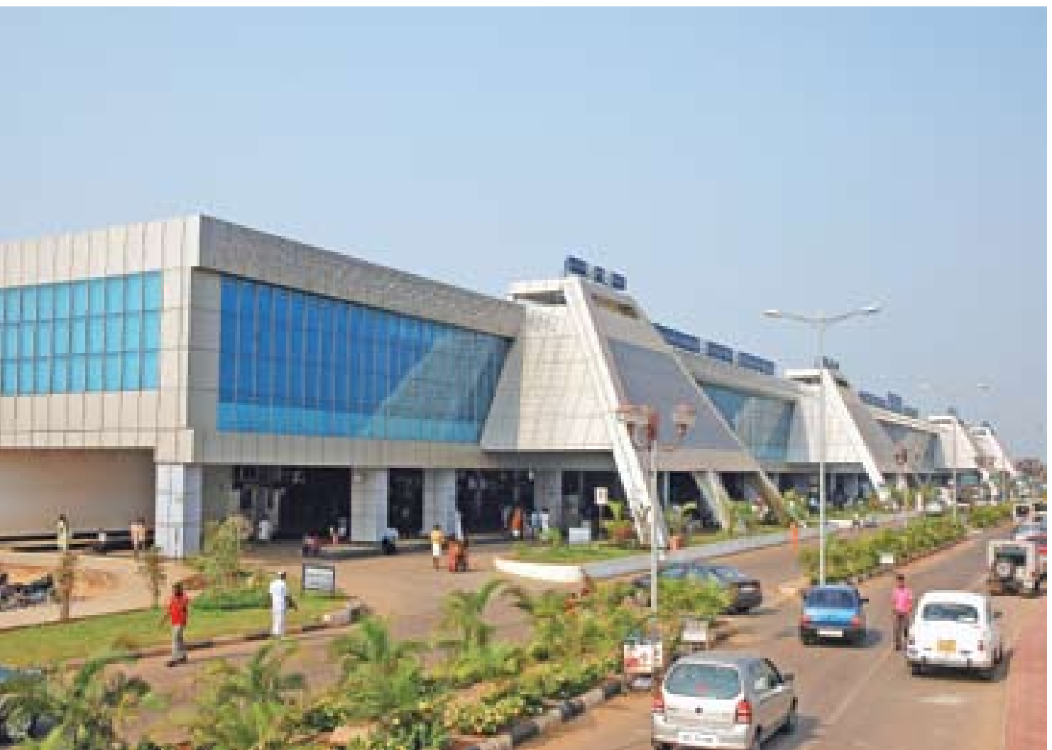
The new Calicut International Airport after renovation.
