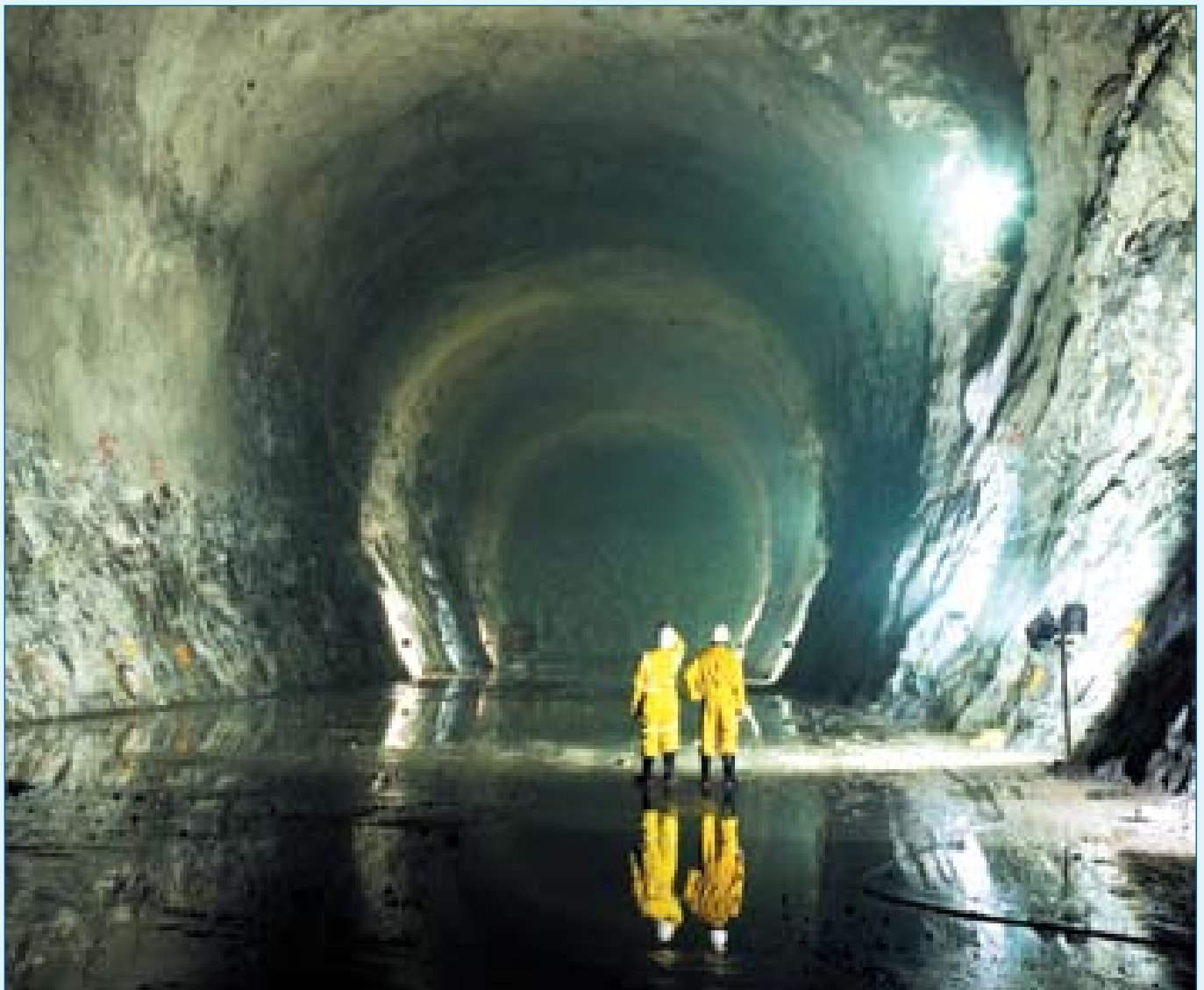
LPG Cavern during construction
