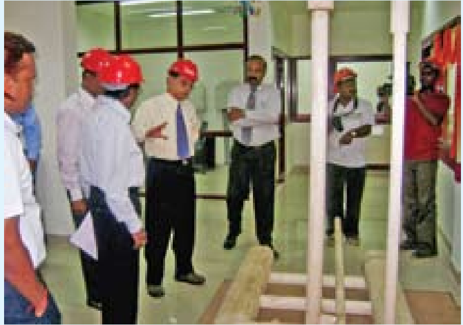
Mr. K.V. Rangaswami, President (Construction) and Member of the Board, L&T, in discussion with ECC colleagues, at the LPG Cavern project, Vizag.
