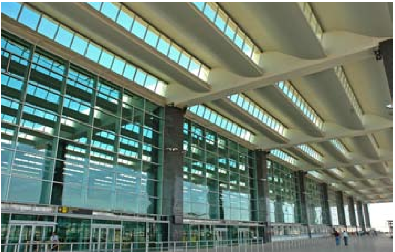
Close-up view of shell roof elements and the glass facade at the entrance to the Passenger Terminal Building
