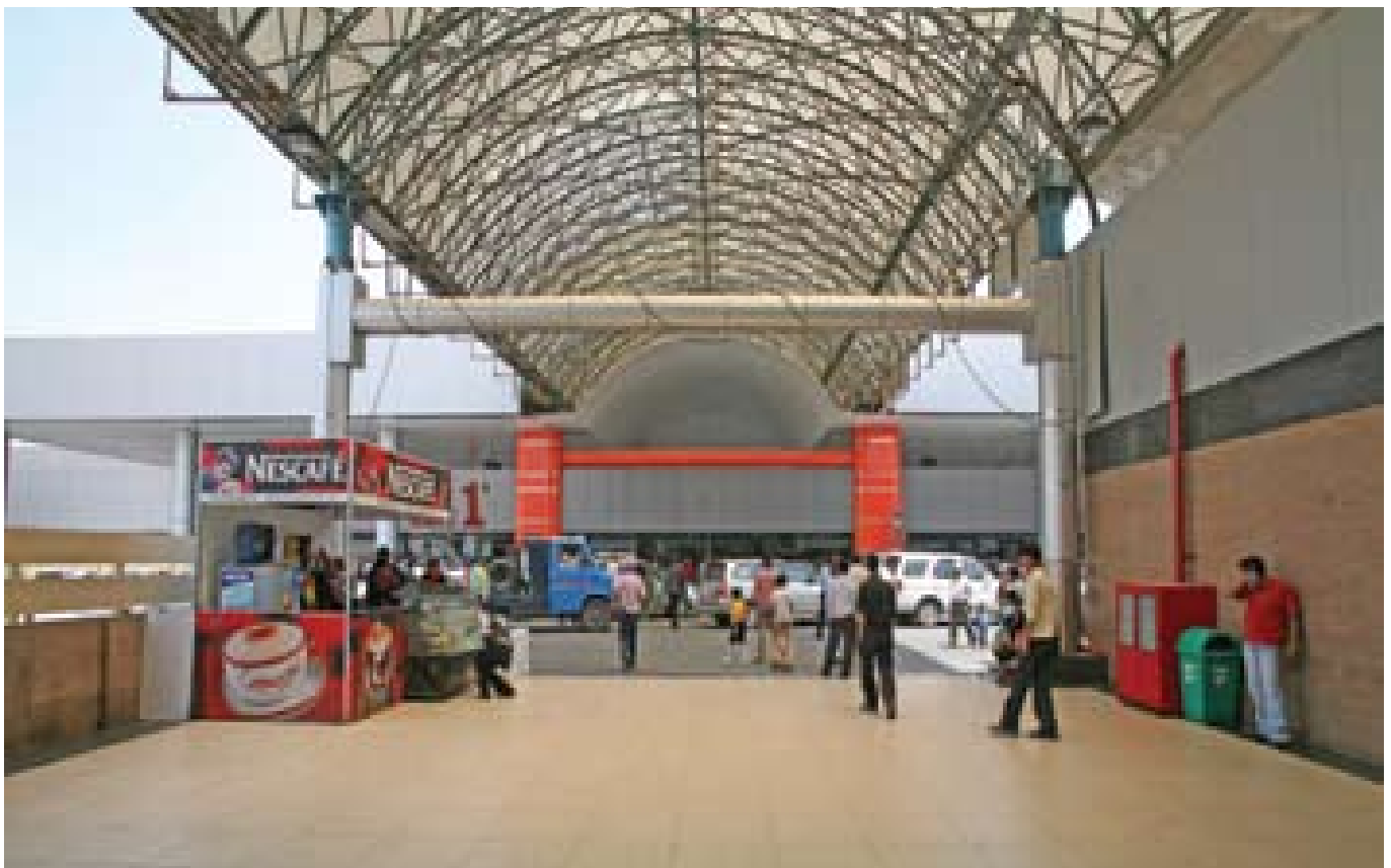
A section of the existing Terminal Building at the Indira Gandhi International Airport, New Delhi
