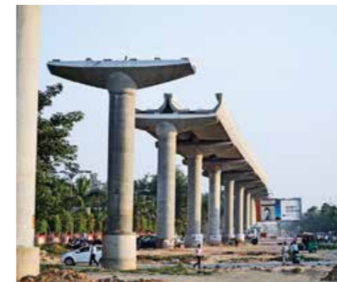
Full span 'U' girder for Delhi Metro
