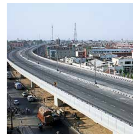
Panipat elevated corridor
