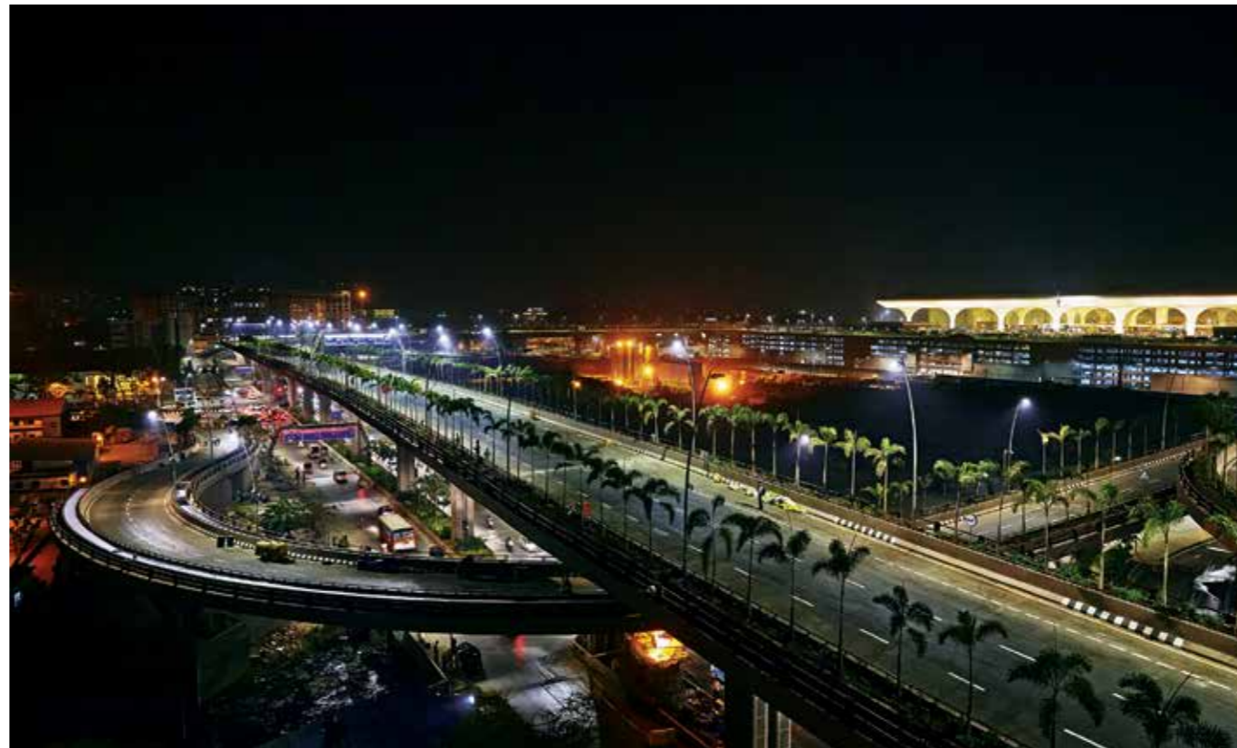
Elevated corridor and forecourt at Mumbai International Airport
