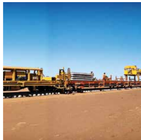
Achieving 2 km track construction per day using mechanized track laying equipment
