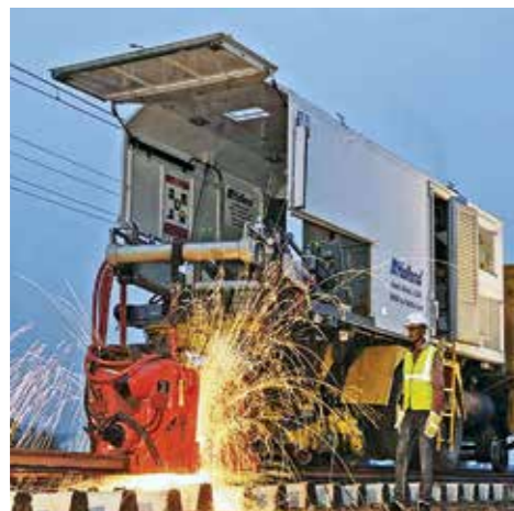
Flash butt welding
