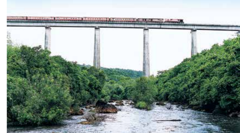
Panvel Nadi viaduct
