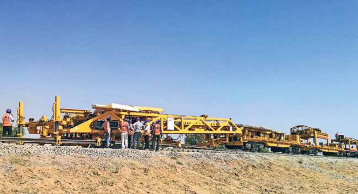
Mechanized track laying
