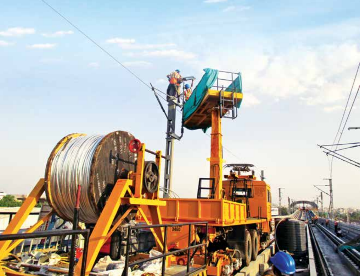
Railway electrification works
