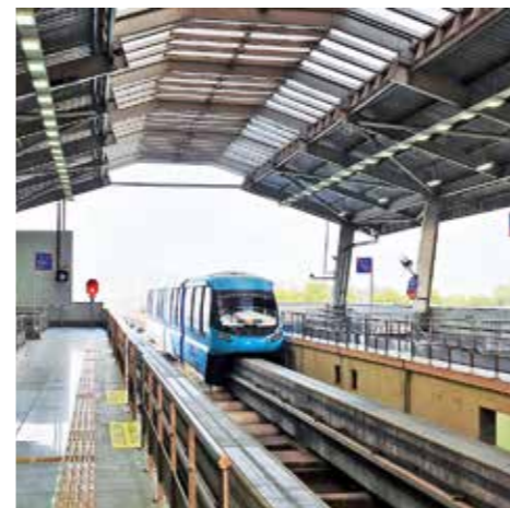
Mumbai Monorail station building
