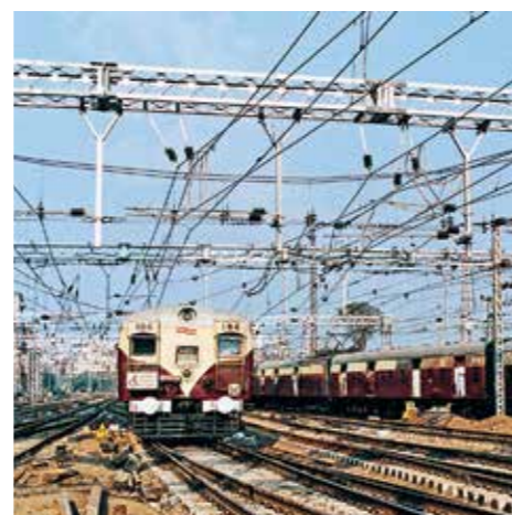
Portal corridors at Mumbai CST yard
