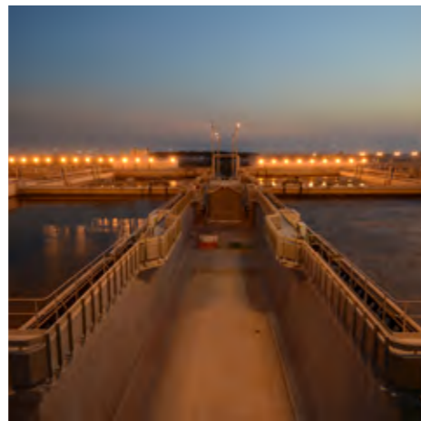
241 MLD Wastewater Treatment Plant, Doha, Qatar
