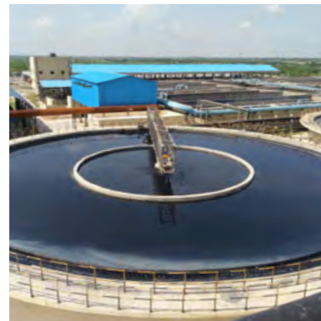
100 MLD Common Effluent Treatment Plant, Narol, Gujarat
