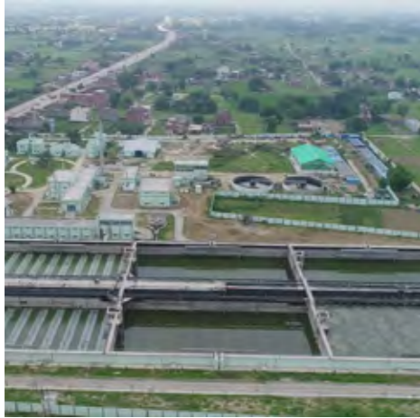
120 MLD Wastewater Treatment Plant, Varanasi, Uttar Pradesh
