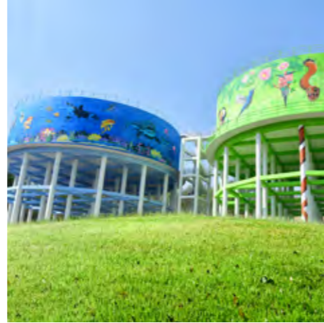
Elevated Storage Reservoir, Pune, Maharashtra
