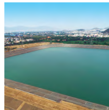
12 Million Cu.m Storage Reservoir for Vizag Steel Plant, Andhra Pradesh
