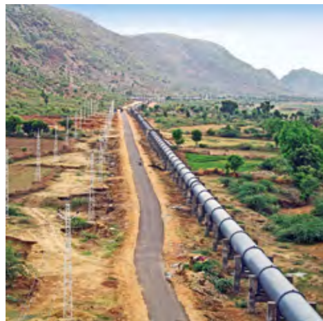
Transmission Mains, Bisalpur, Rajasthan
