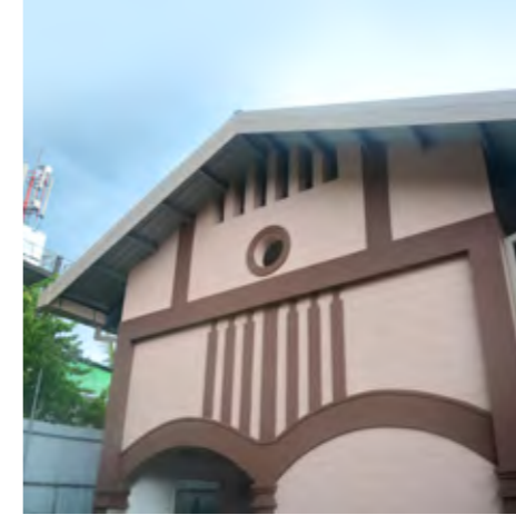
Rehabilitation of Wastewater Pumping Stations for Colombo Municipal Council, Sri Lanka
