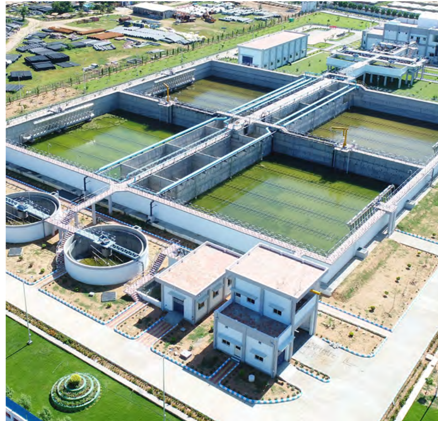
55 MLD Wastewater Treatment Plant, Nellore, Andhra Pradesh
