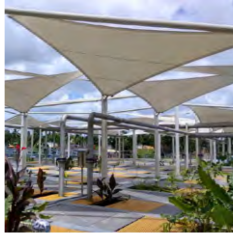
31 MLD Wastewater Treatment Plant, Bhatpara, West Bengal
