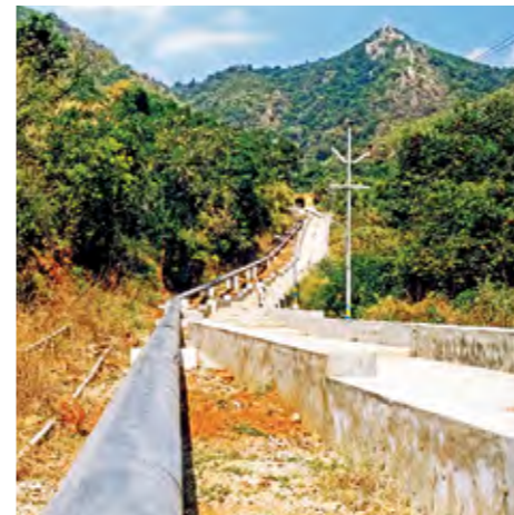
Pipeline installed on steep gradients
