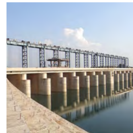
Kharkai Barrage, Jharkhand
