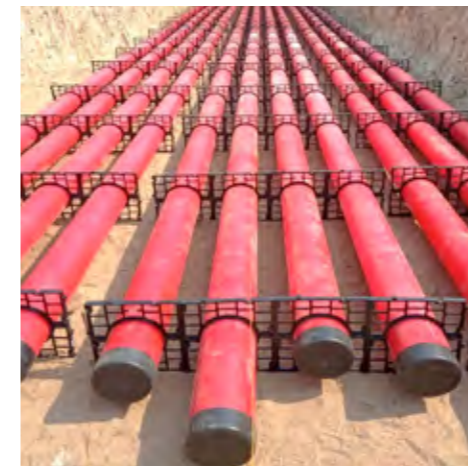
PLB Duct at Amaravati, Andhra Pradesh
