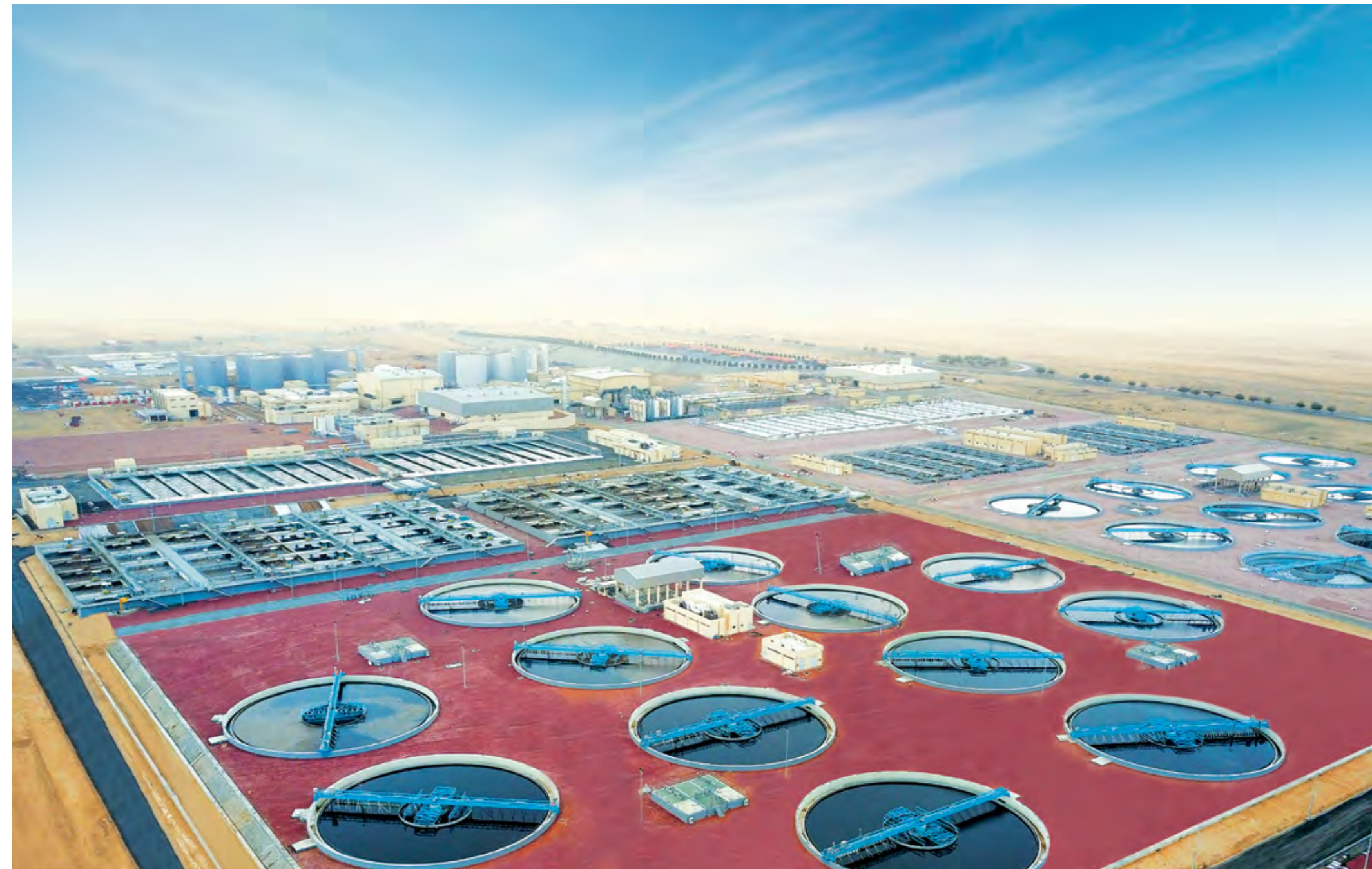
375 MLD Wastewater Treatment Plant, Jebel Ali, UAE
