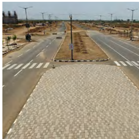
Green-field development at Dholera, Gujarat
