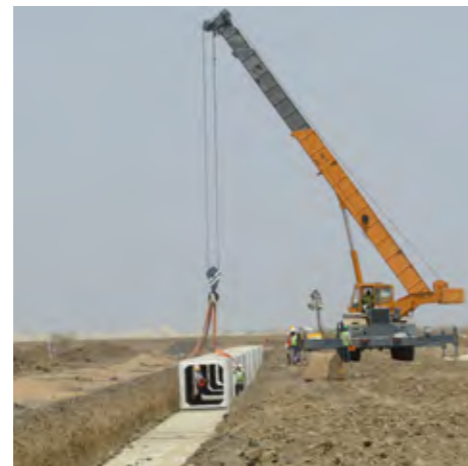
Precast duct laying at Amaravati, Andhra Pradesh
