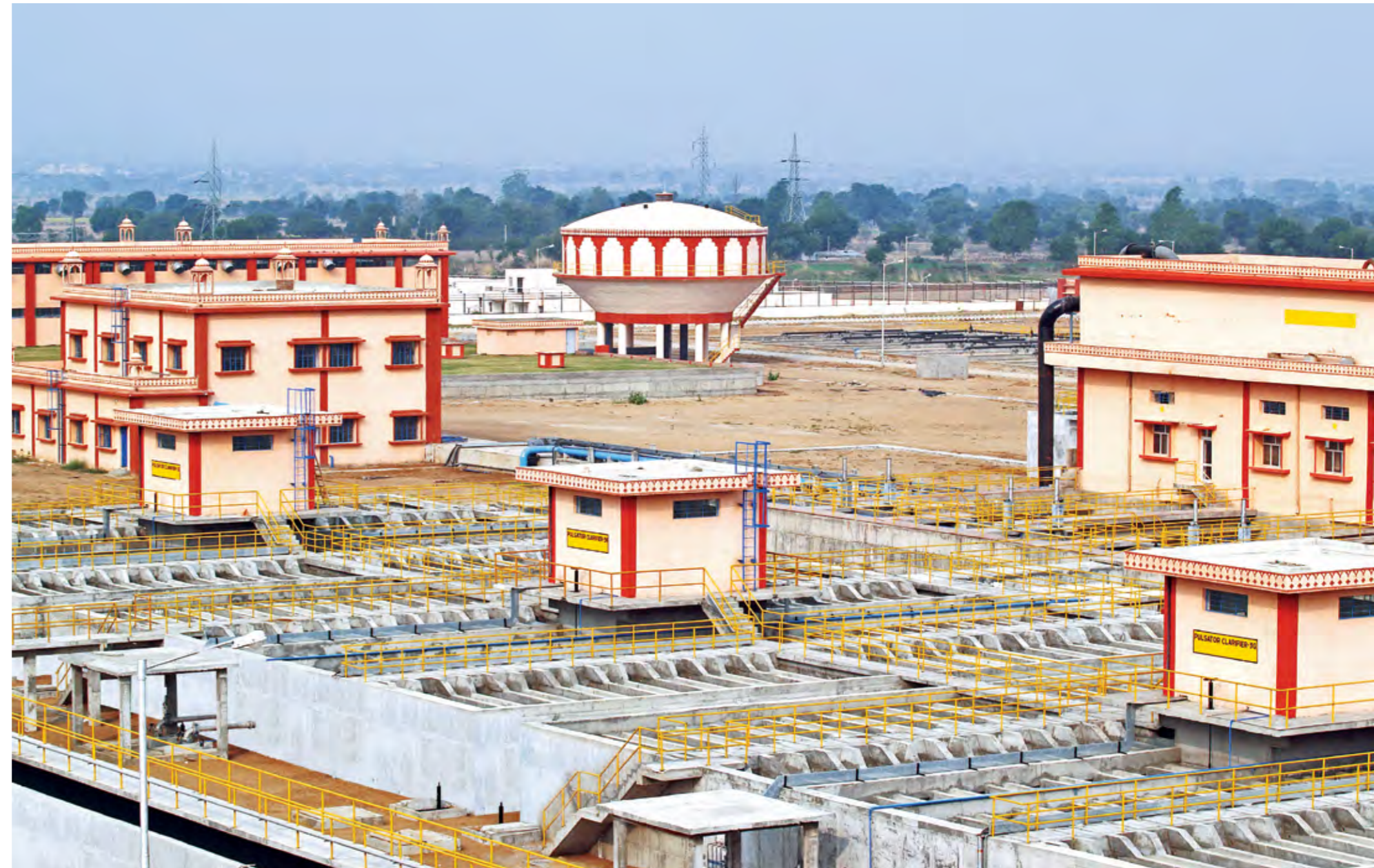
Bisalpur-Jaipur Water Supply Scheme with 400 MLD WTP, Rajasthan
