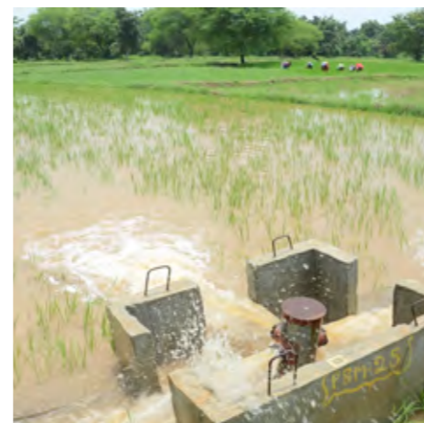
Delivery Chamber for a Mega Lift Irrigation Project, Odisha
