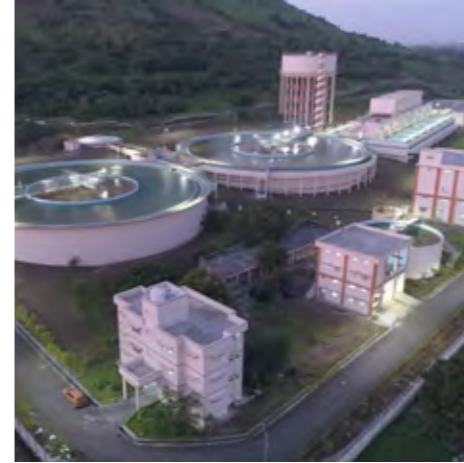
137 MLD Water Treatment Plant at Nashik, Maharashtra
