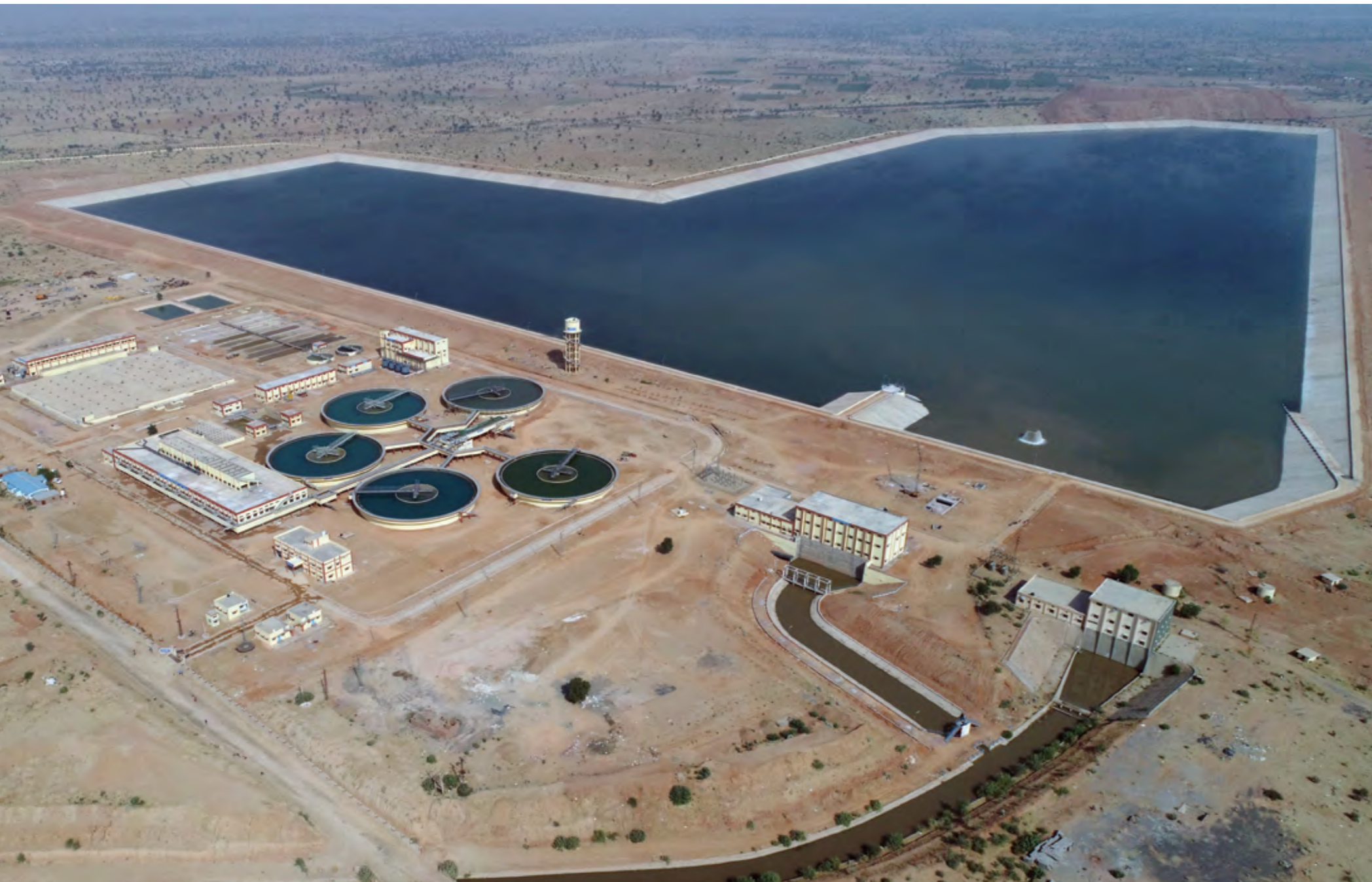
Aerial view of the 250 MLD Water Treatment Plant and 5310 ML Raw Water Reservoir, Nagaur, Rajasthan
