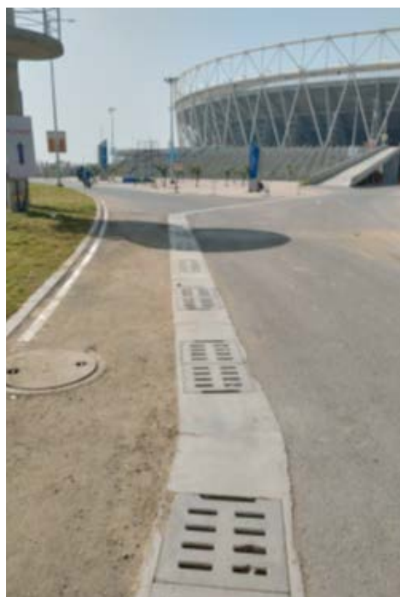
Storm water system - Post construction
