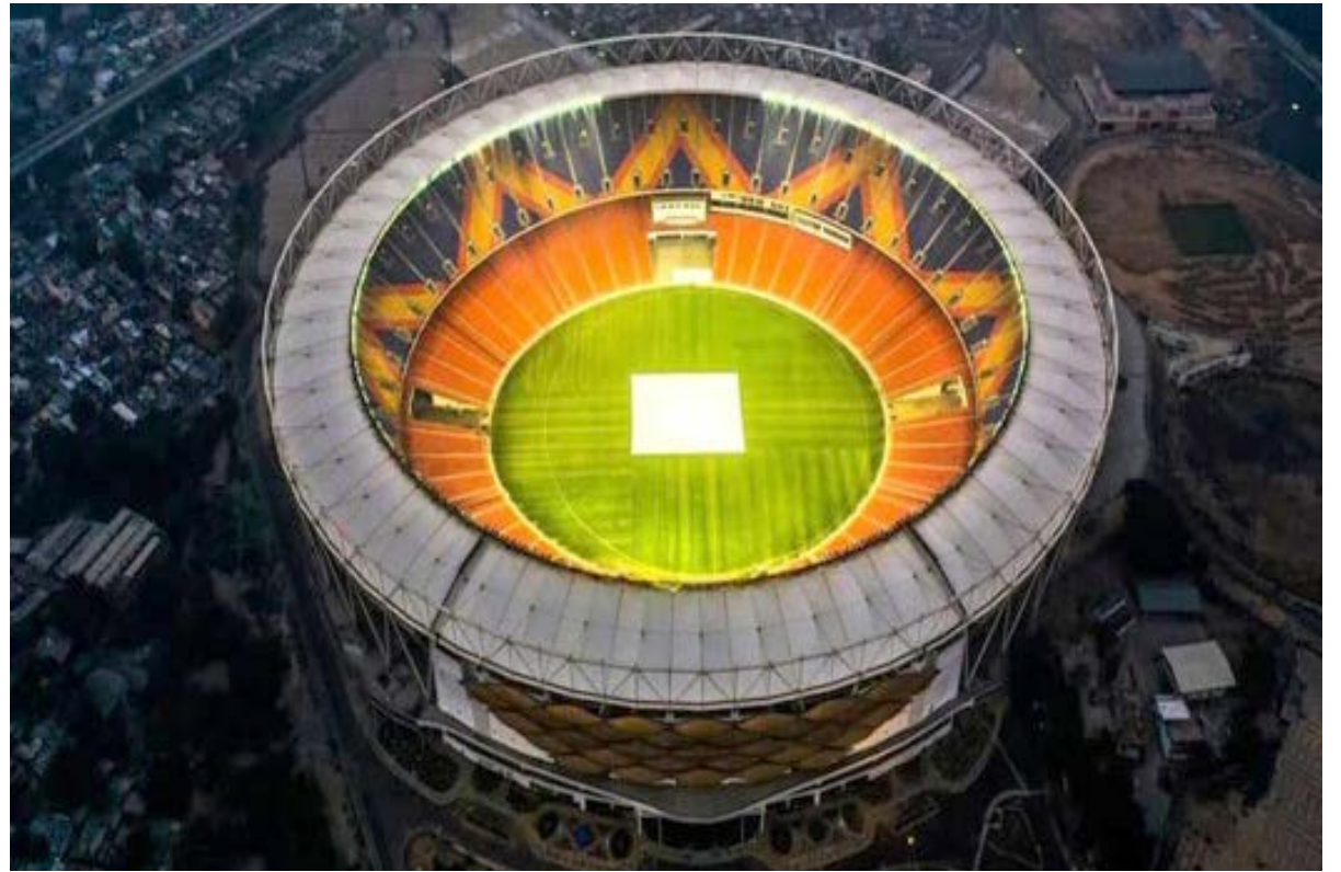
Stadium FOP (Field of Play) lighting
