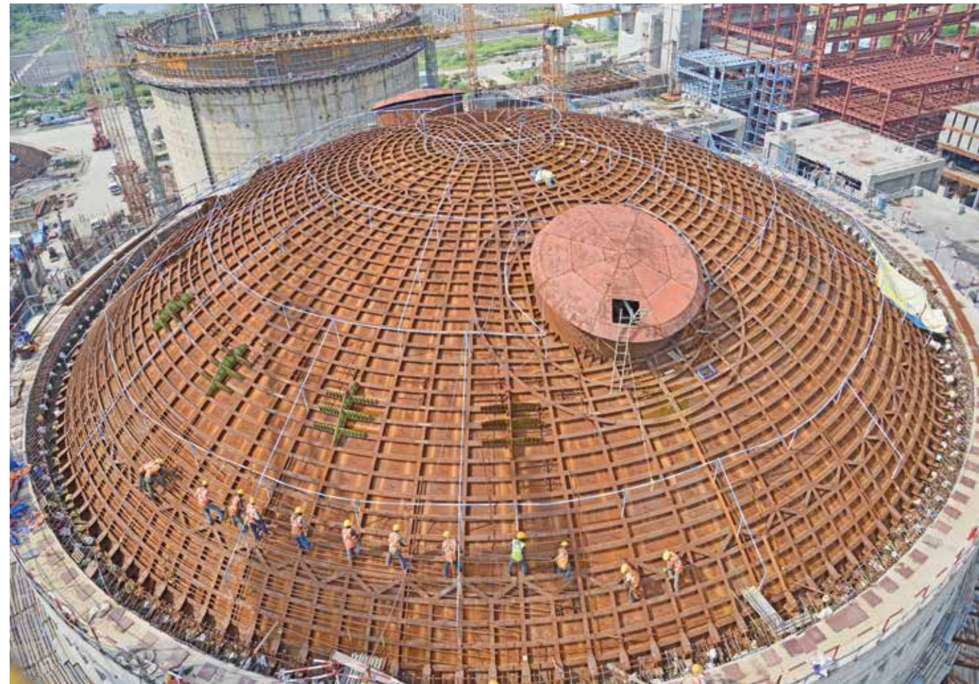
Workmen fixing the individual panels of the prefabricated ring liner
