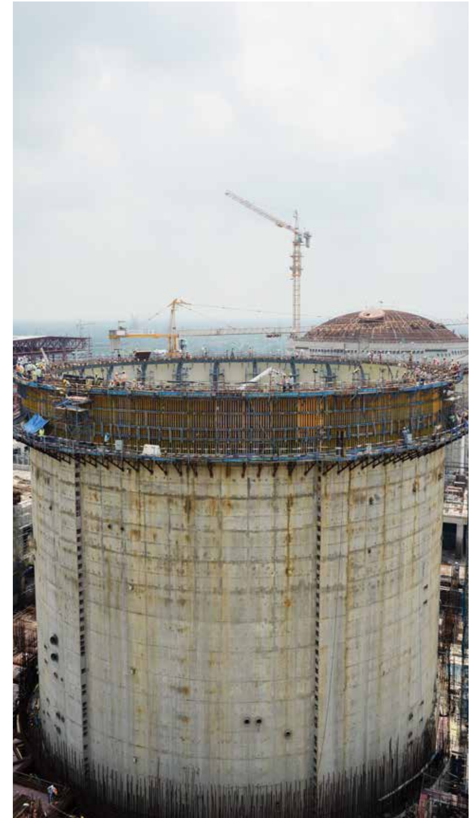
Construction of the reactor building in progress
