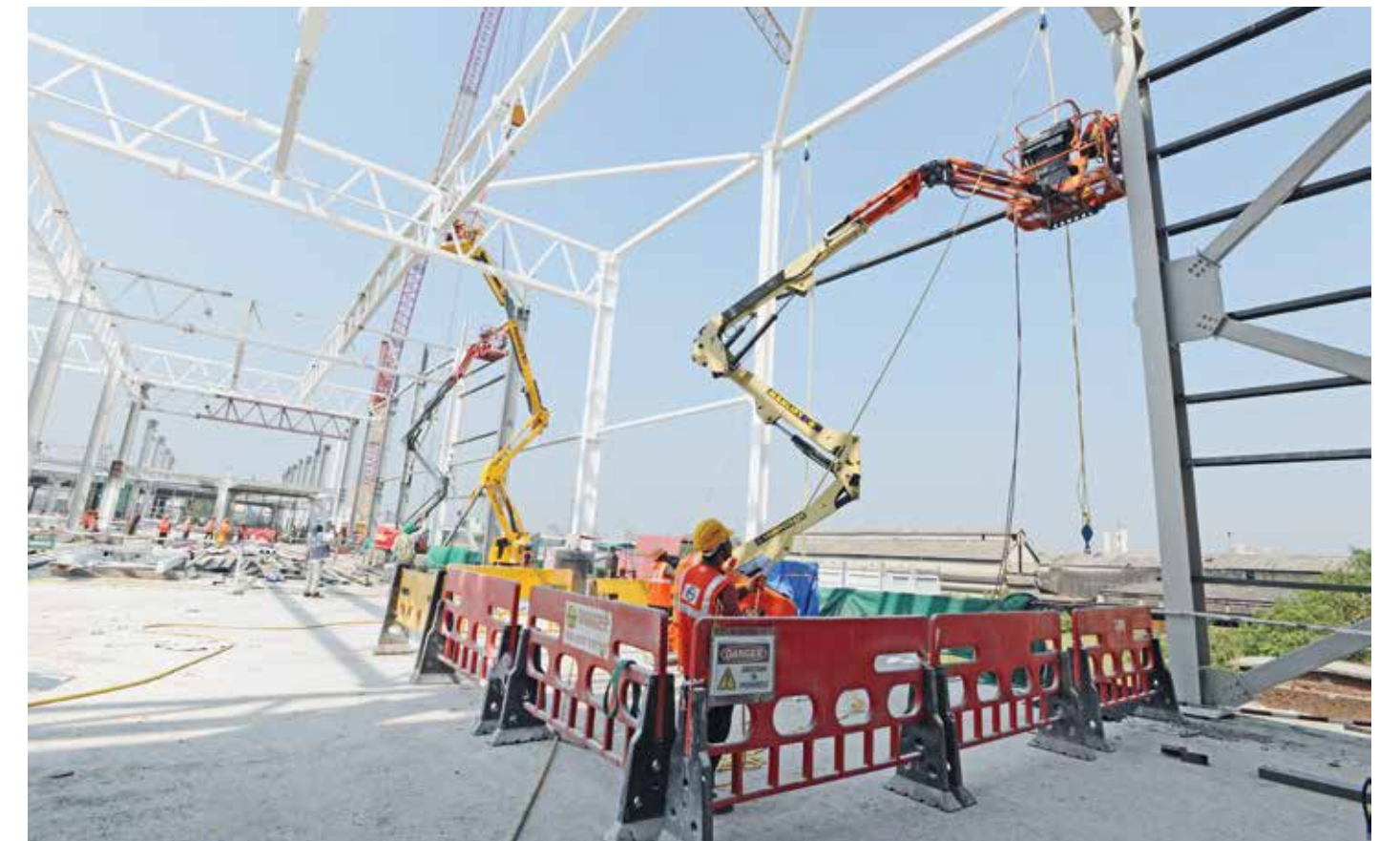
Erection of structural steel
