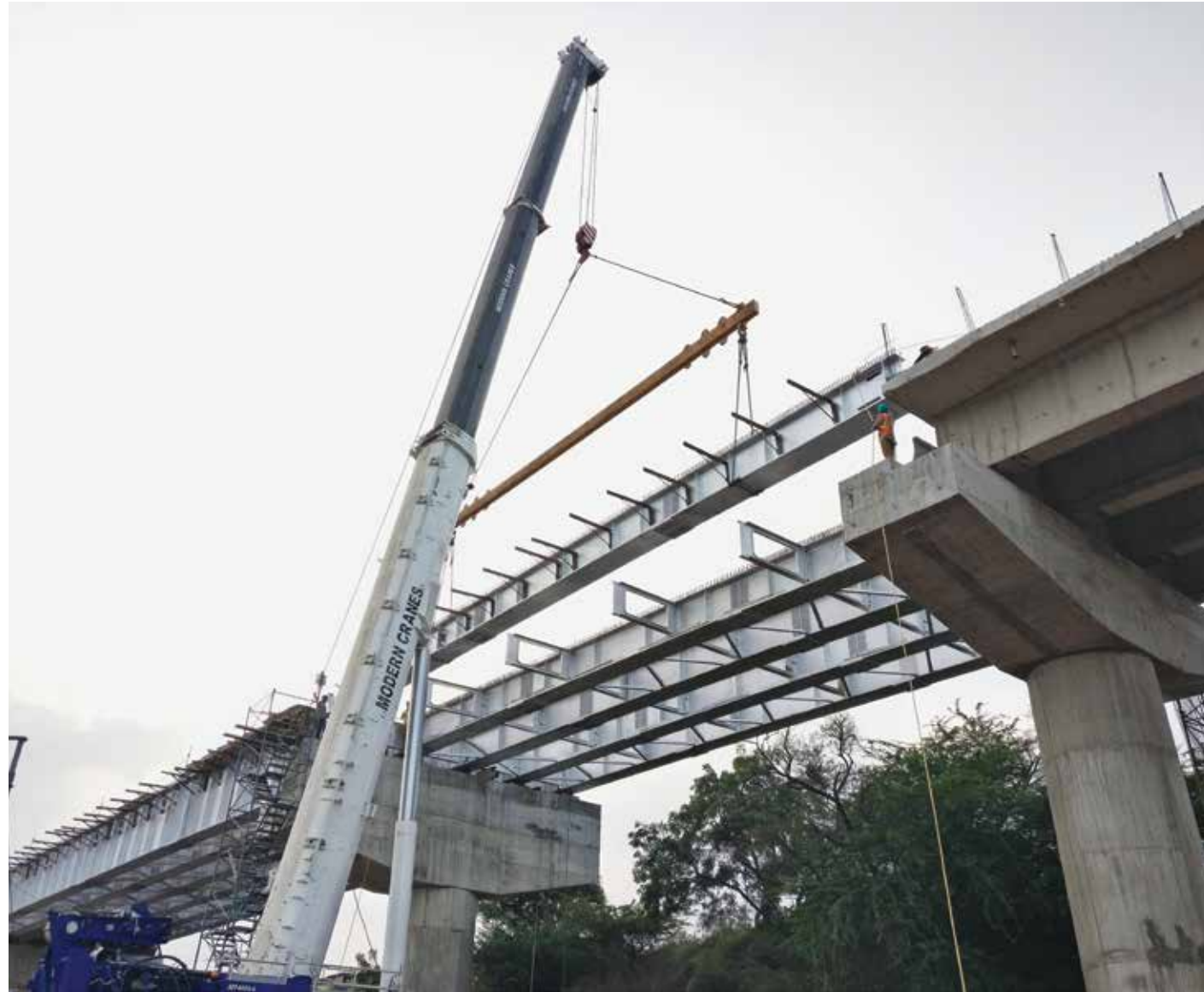
Steel girder erection
