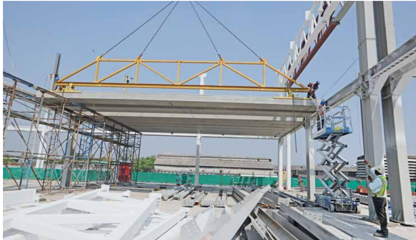
Hollow core erection
