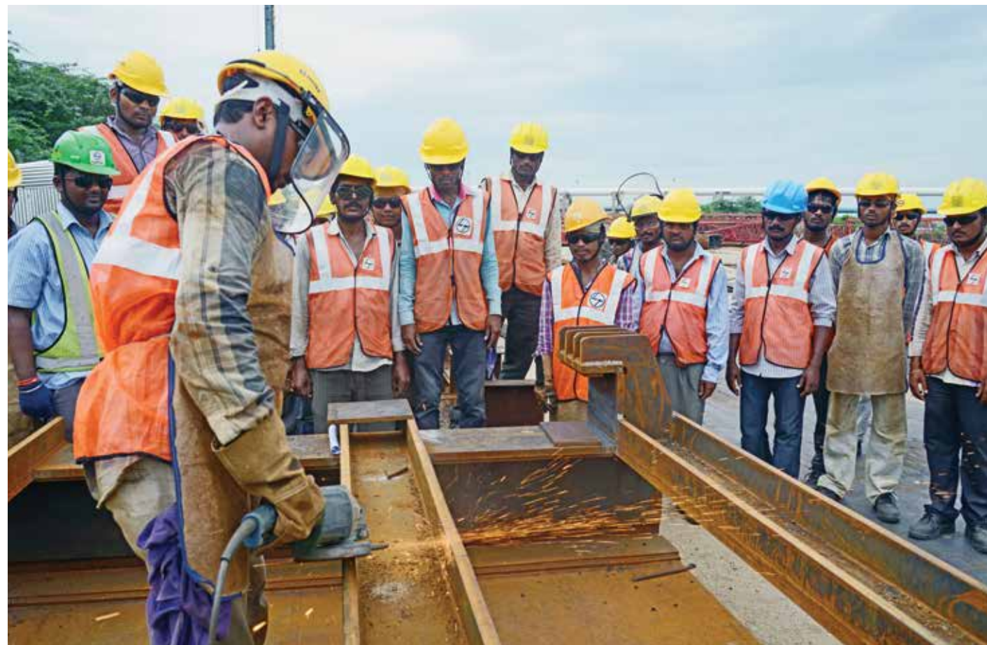
Welding demonstration to workmen
