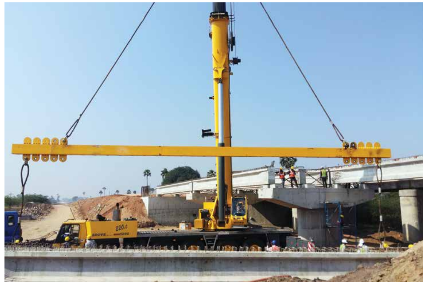
RCC girder erection
