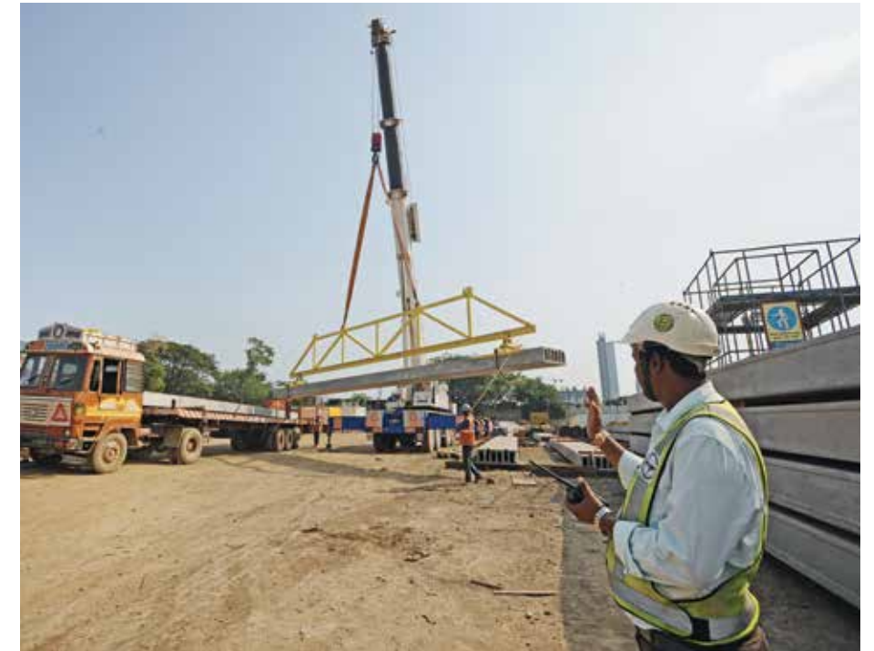
Hollow core handling
